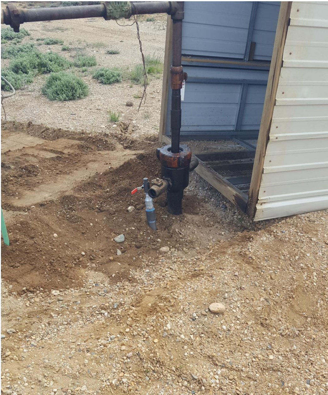
Figure #1 Bradenhead access has been installed.
