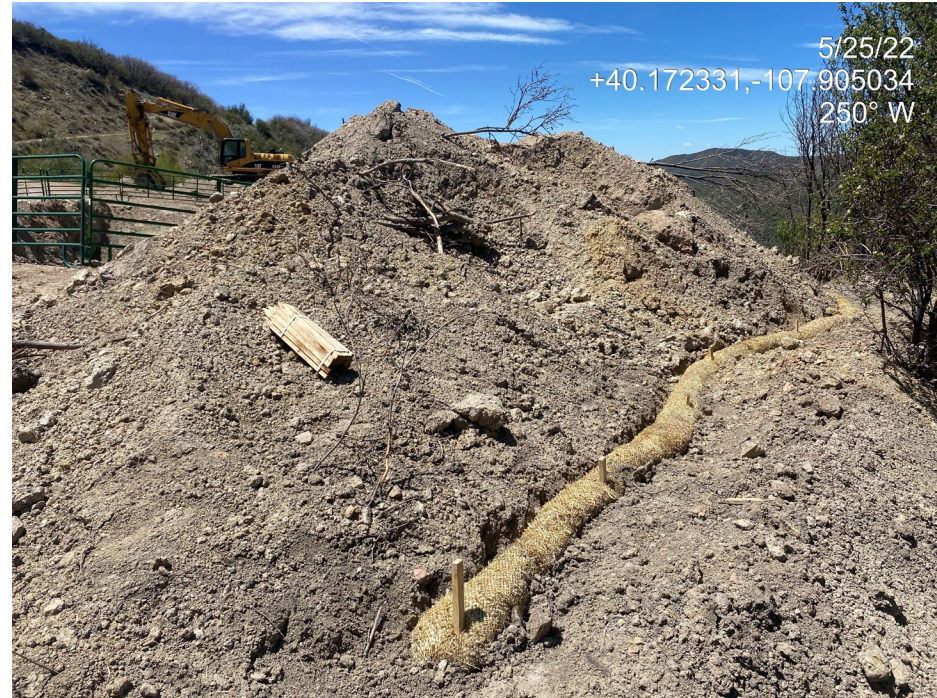
Photo 2. Photo taken from the east of the Location shows a soil pile. A straw wattle has been added around the downslope perimeter of the pile.
