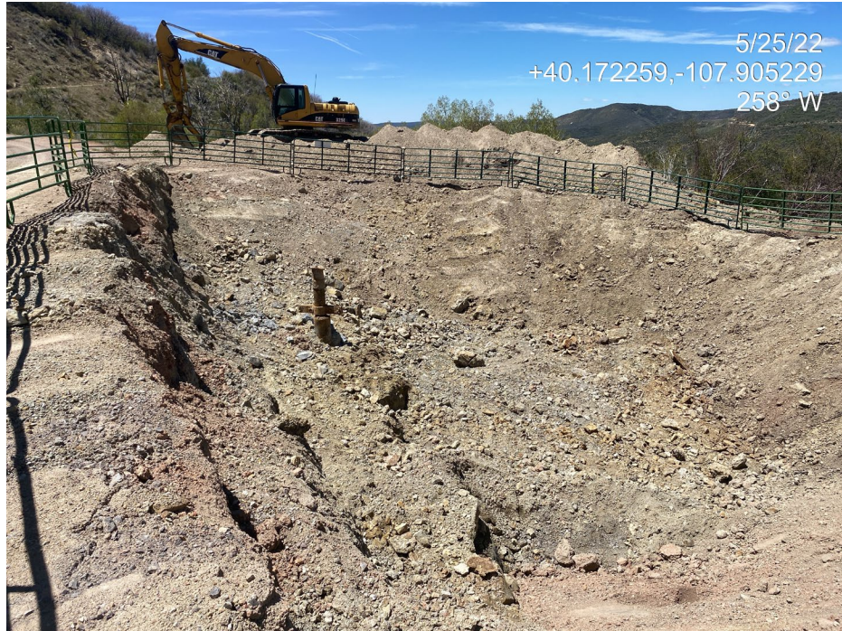
Photo 1. Photo taken from the well area shows the excavation around the wellhead. The slope of the sides is gentle enough to allow for wildlife egress. Fence panels are present around the entire excavated area.
