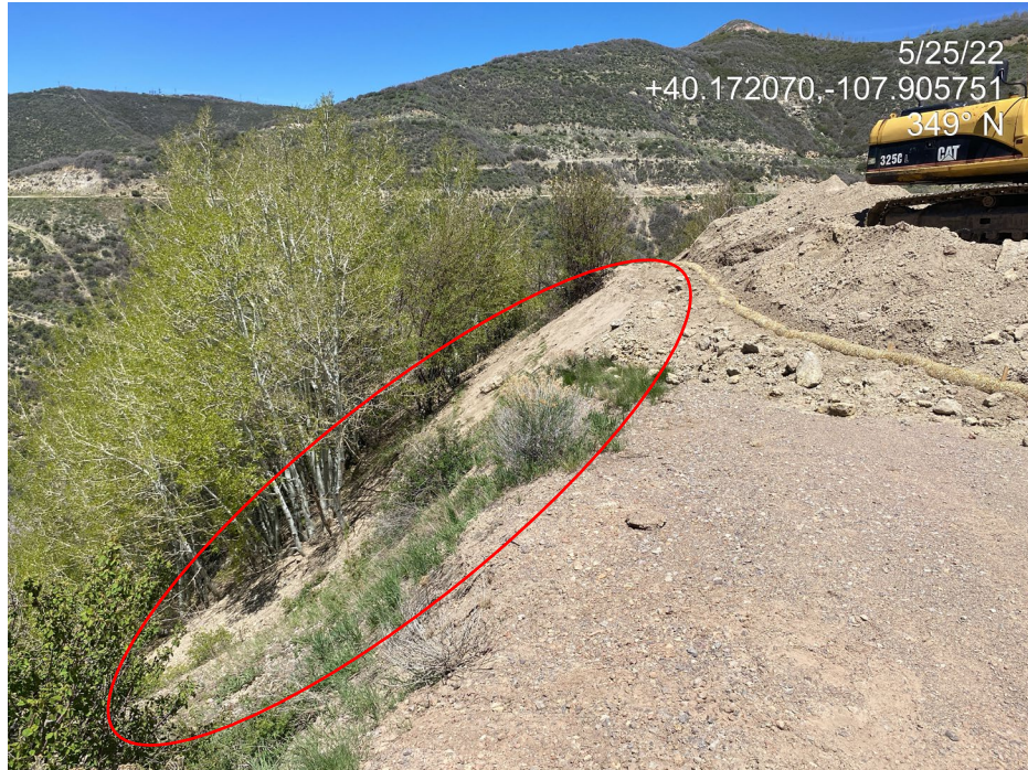
Photo 3. Photo taken from the west of the Location shows a soil pile to the right. A straw wattle has been added around the downslope perimeter of the pile. Piles of soil from the Location are present downslope of the wattle and off site.
