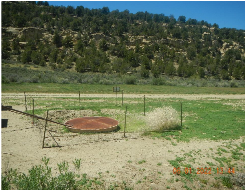
Fence around pit is broken and fallen.
