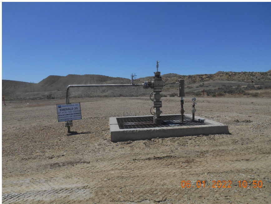
Injection wellhead.
