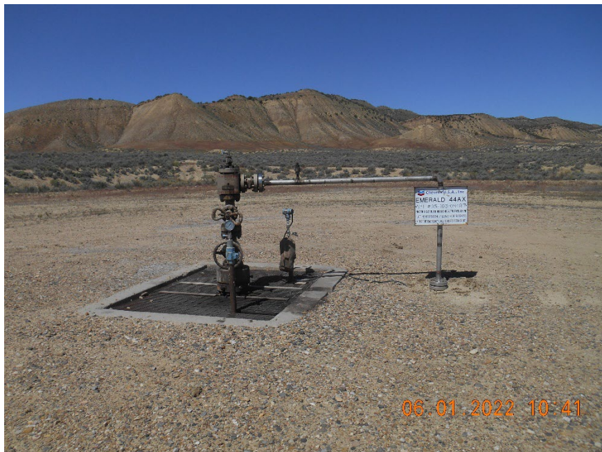
Injection wellhead.
