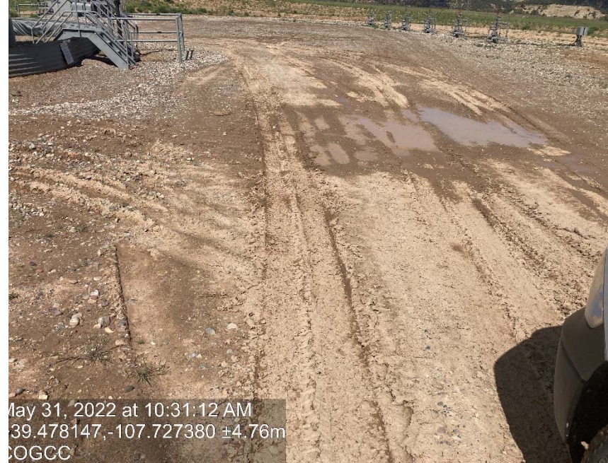
Lack of stabilization/ compaction/ degradation
