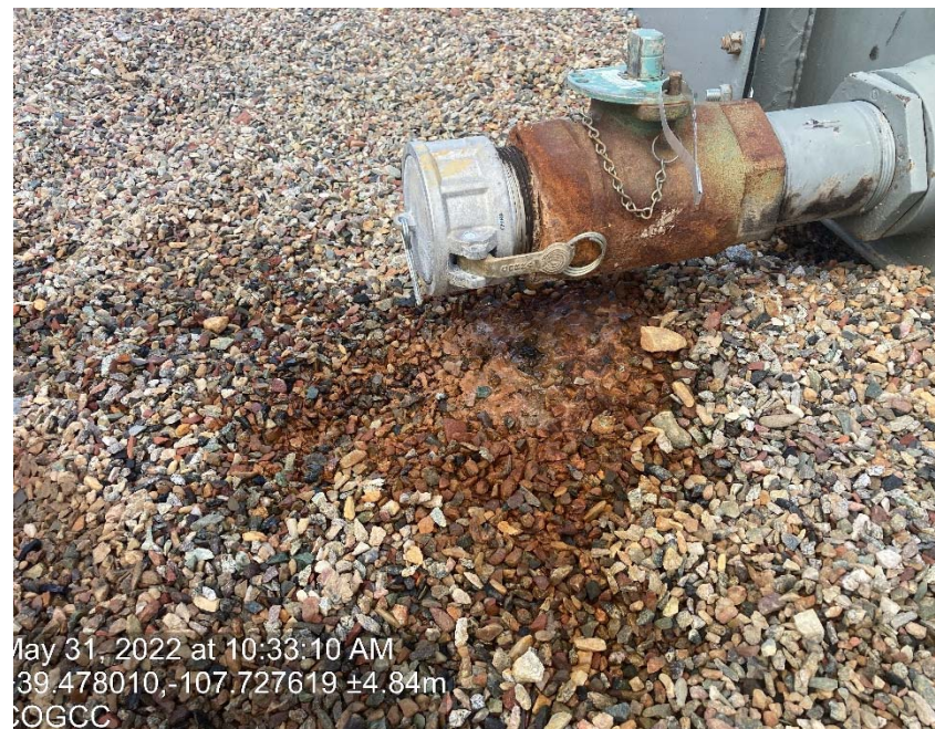
Valve leaking
