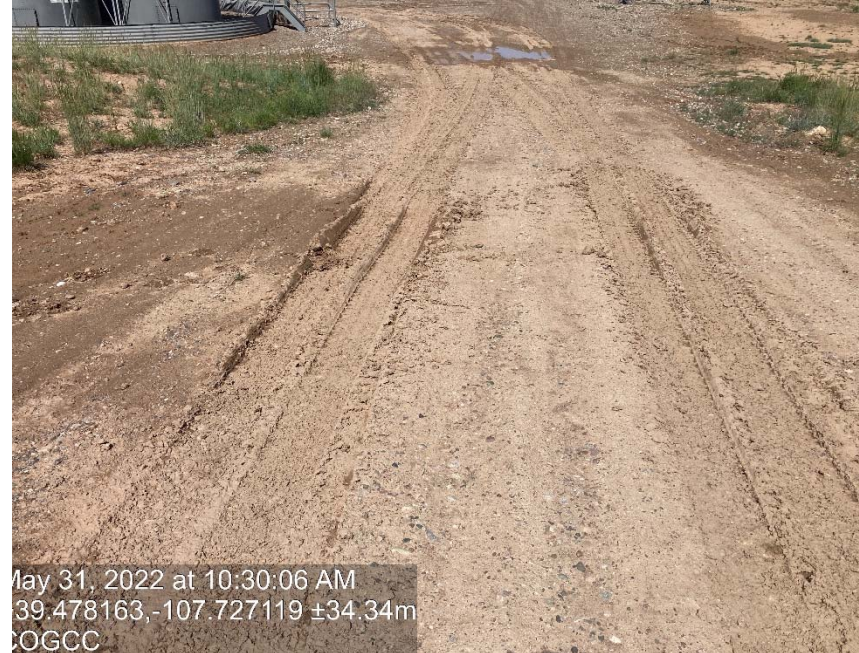
Lack of stabilization/ compaction/ degradation
