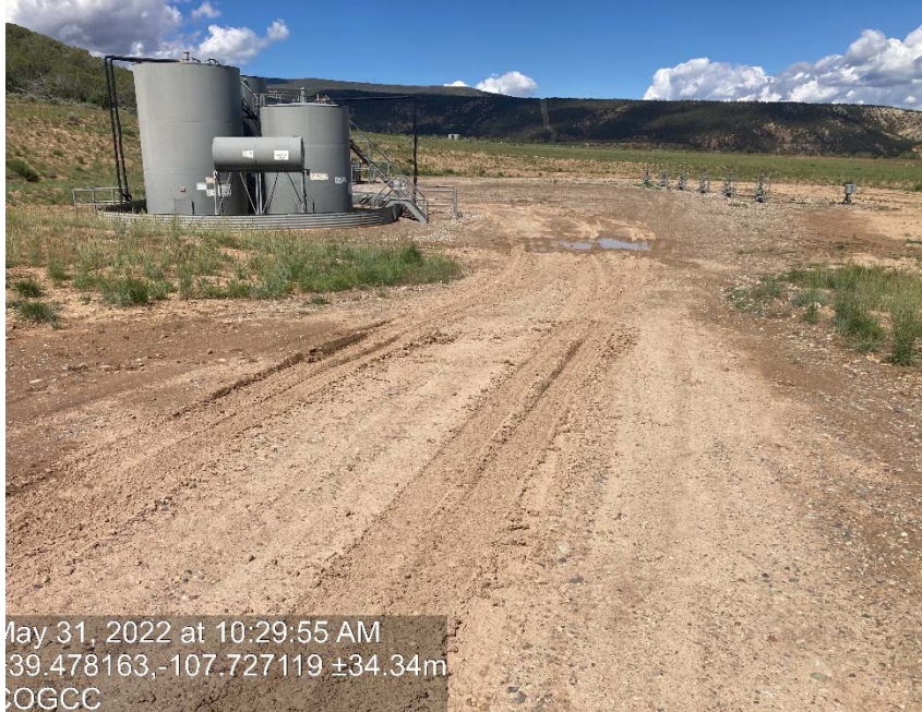
Lack of stabilization/ compaction/ degradation
