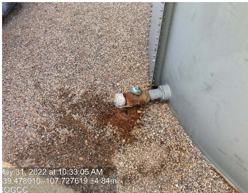
Valve leaking
