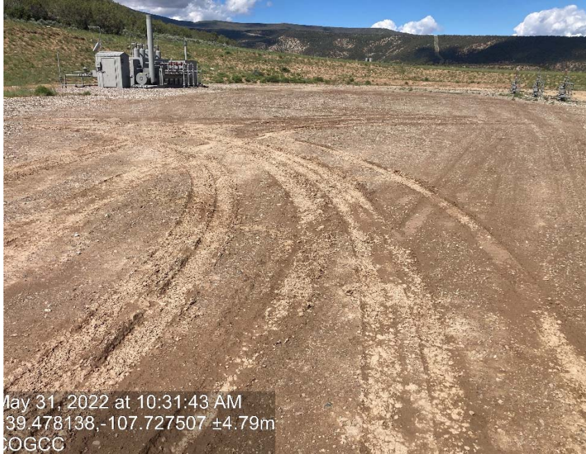
Lack of stabilization/ compaction/ degradation
