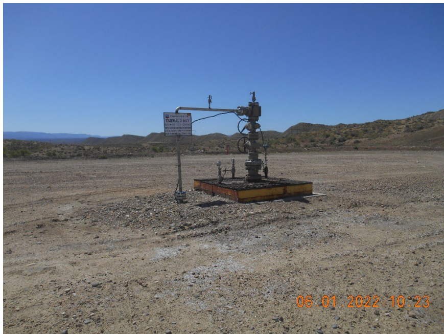
Injection wellhead
