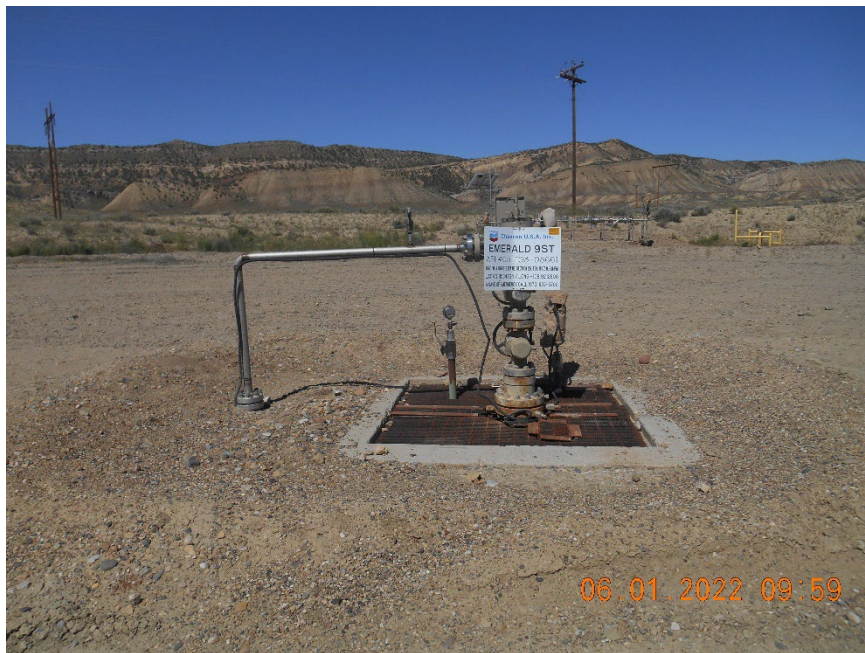
Injection wellhead
