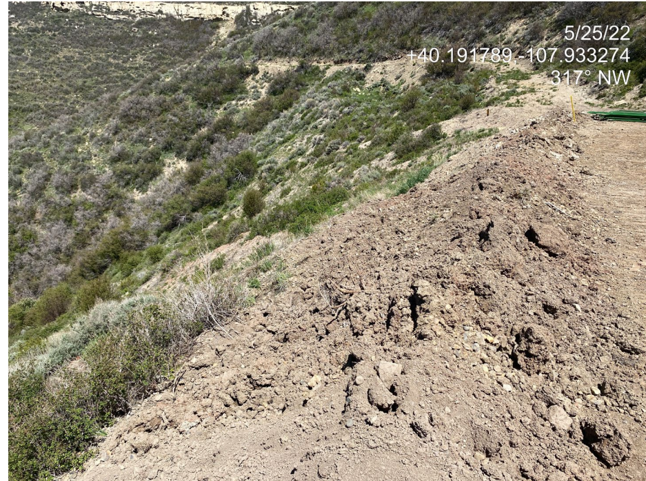
Photo 4. Photo taken from the west of the Location shows a soil berm at the edge of the Location intended as a temporary measure to prevent migration of E&P waste off site. The berm may act as a sediment source/stormwater pollutant.
