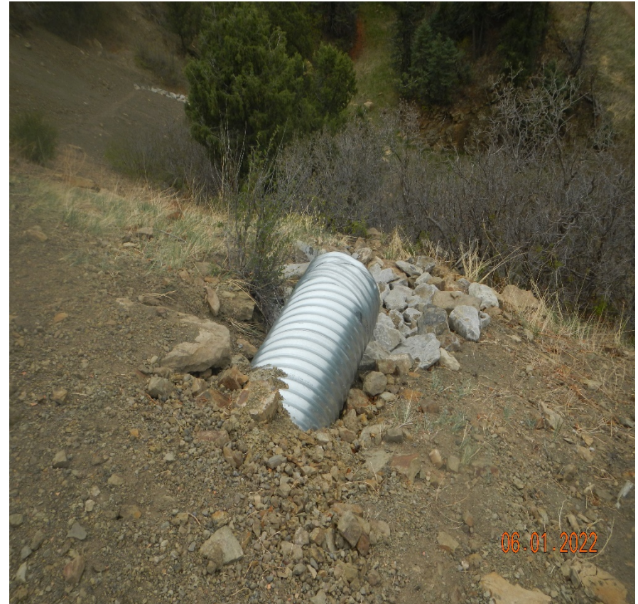
Photo 4. A new culvert has been installed with outlet protection.
