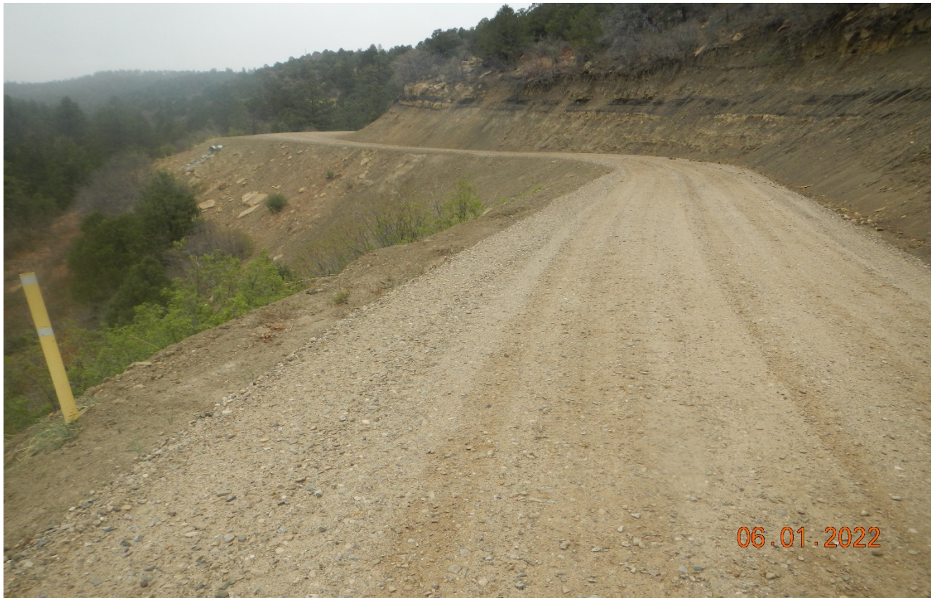
Photo 2. Facing west. The road sides has been regraded and erosion repaied.
