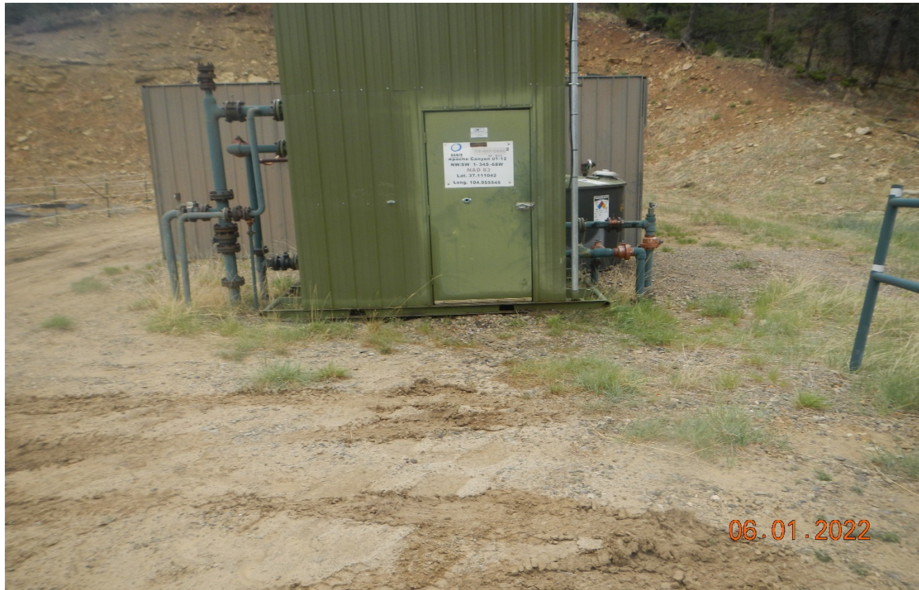
Photo 7. The leak at the shed was repaired and cleaned up.
