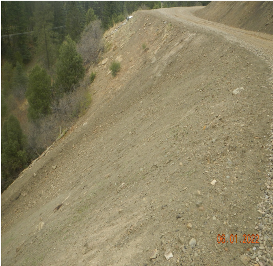
Photo 3. The slope of the road side was regraded and seeded. A berm was installed at the toe of slope. This area needs to be monitored for stabilization and may require additional BMP's.
