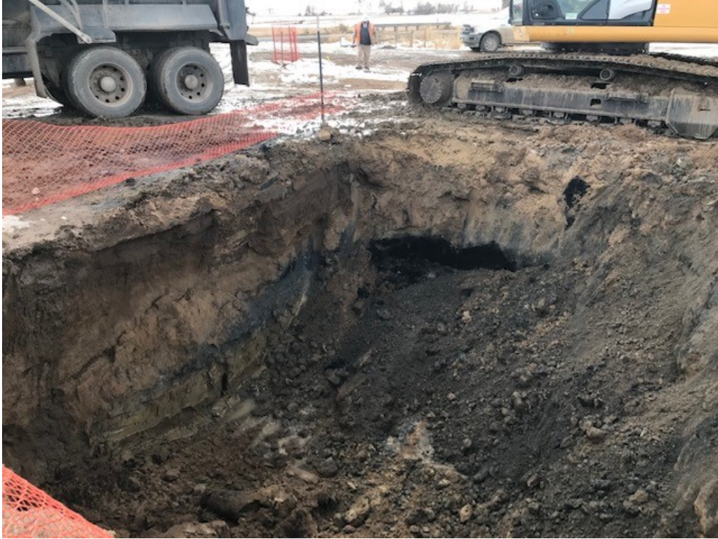
#5 – Looking Southwest at Excavation
