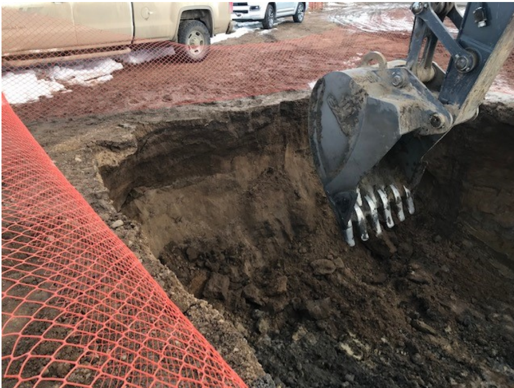
#6 – Looking Southeast at Excavation
