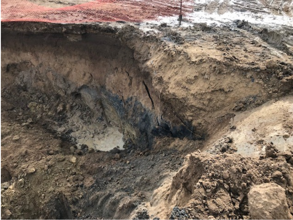
#1- South Wall of Former Produced Water Vault
