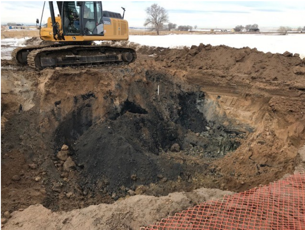
#4 – Looking Northwest at Excavation
