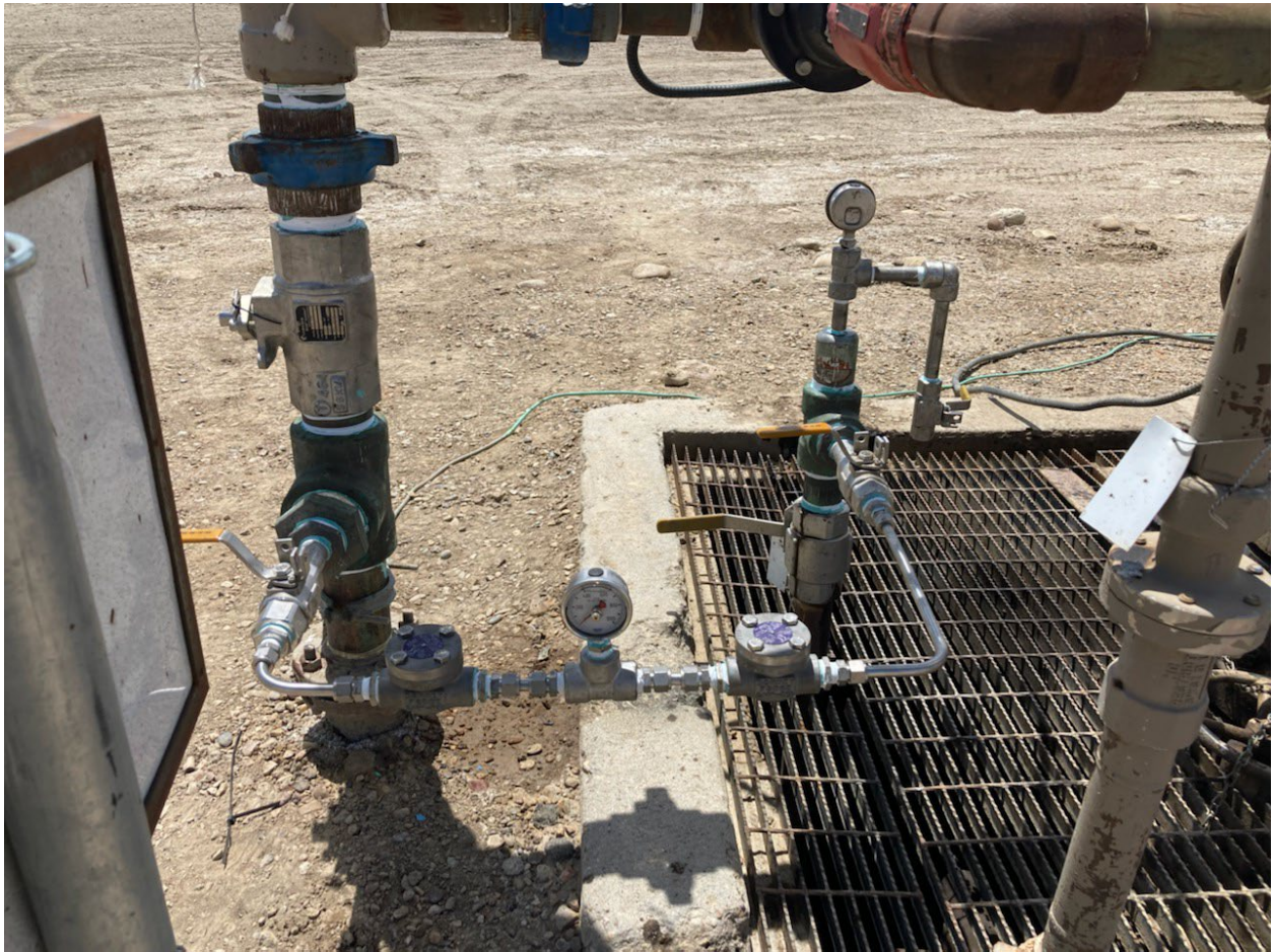
Fee 82X Bradenhead piping installed
