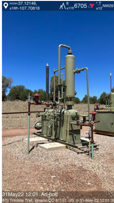
IMG 07 Vertical Separator
