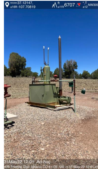
IMG 08 Vertical Separator
