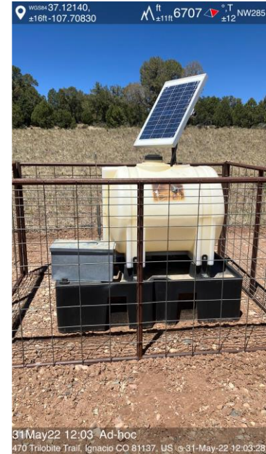
IMG 12 Scale corrosion inhibitor sign is deteriorated and NFPA sign is illegible
