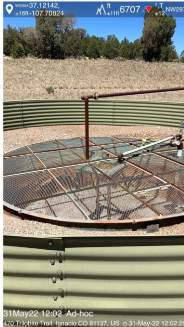
IMG 11 Produced water tank
