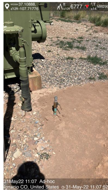
IMG 22 Unused flow line
