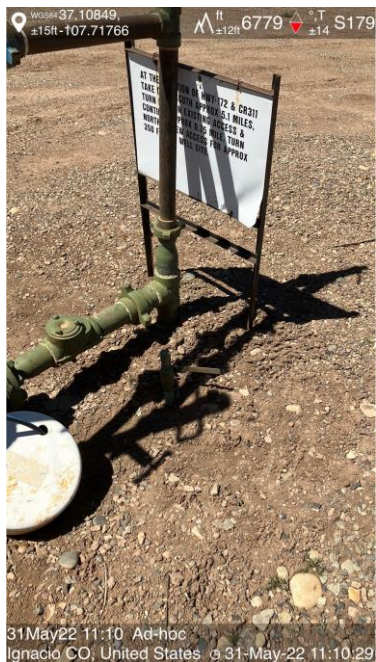
IMG 23 Unused flow line
