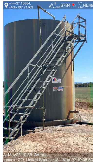
IMG 12 Produced water tank
