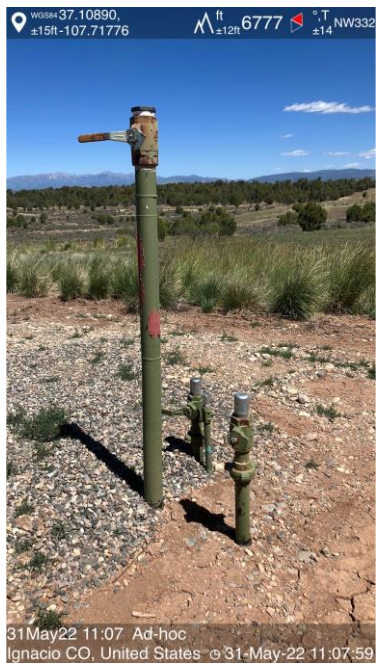
IMG 21 Unused flow lines
