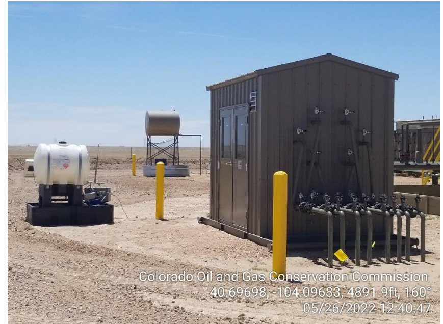
Photo 6 – Gas Lift Injection Meter House
