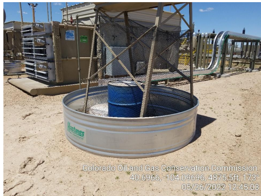
Photo 18 – Wildlife Netting is missing/disrepair
