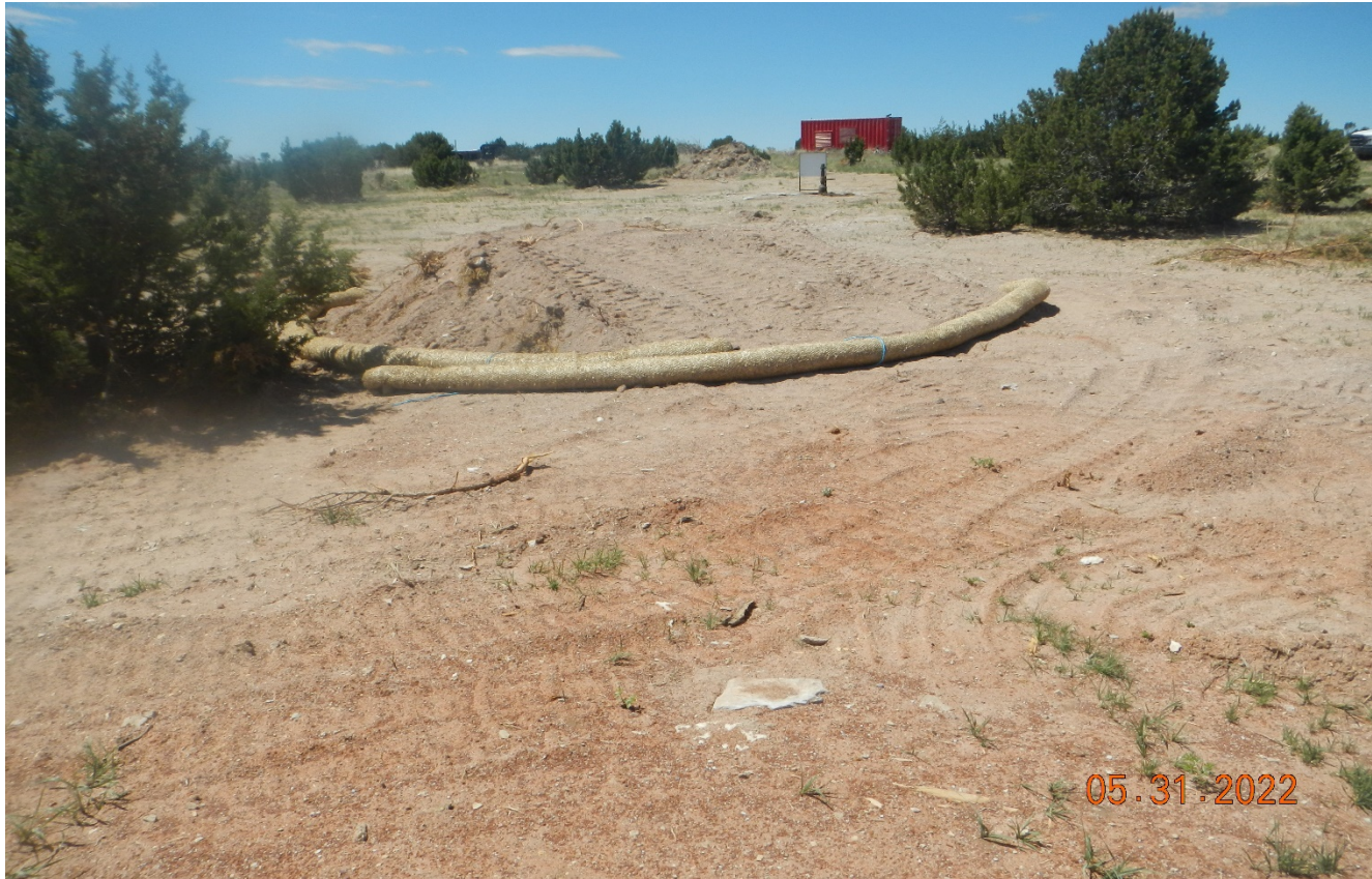
Photo 7. It is unknown which pile of material is the cuttings pile. It appears some cuttings is on the surface in photo. The wattles are not staked down around the pile.
