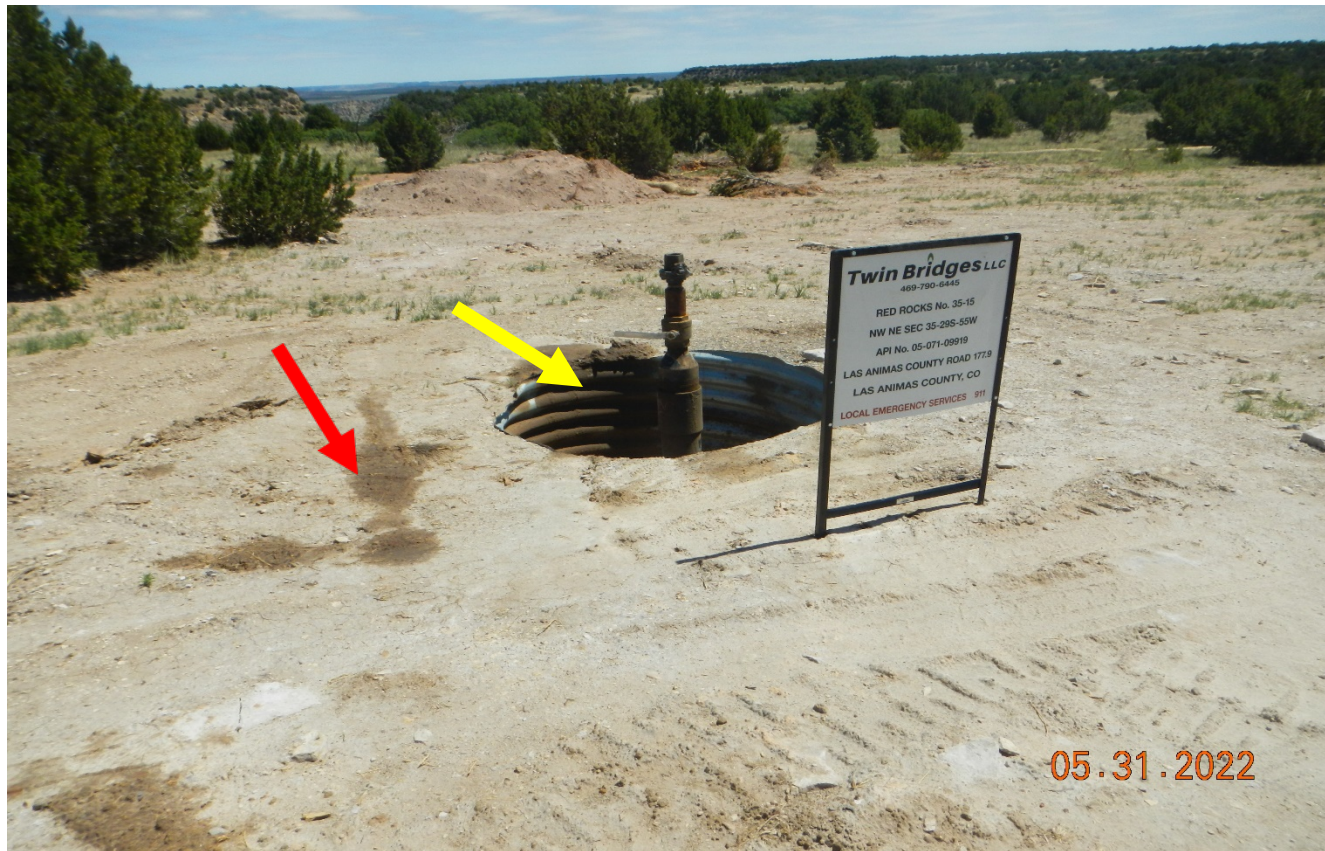
Photo 4. The well has been drilled at the location. The wellhead cellar (yellow arrow) needs to be covered to prevent entry. There is oil stained soils (red arrow) that need to be cleaned up.
