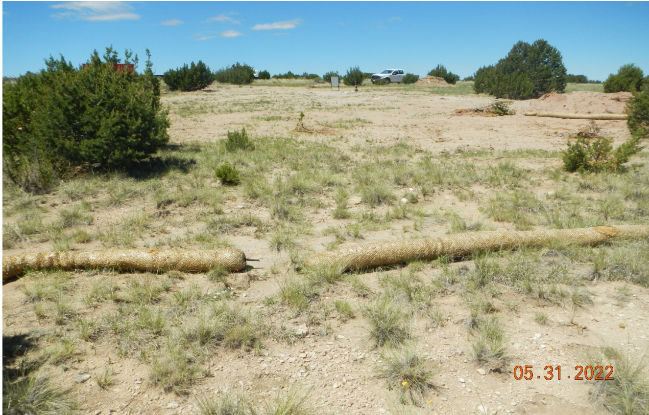
Photo 5. The down gradient straw wattles are not installed correctly. There is a gap between the ends of the wattles and there is no staking to hold them in place.
