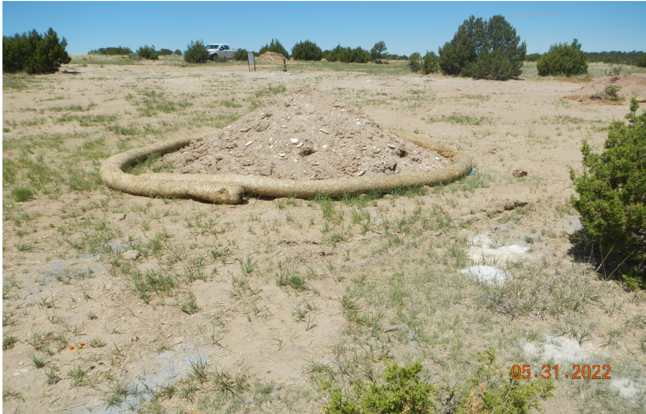
Photo 8. There are a multiple soil piles around the location. The wattles are not staked down around the pile.
