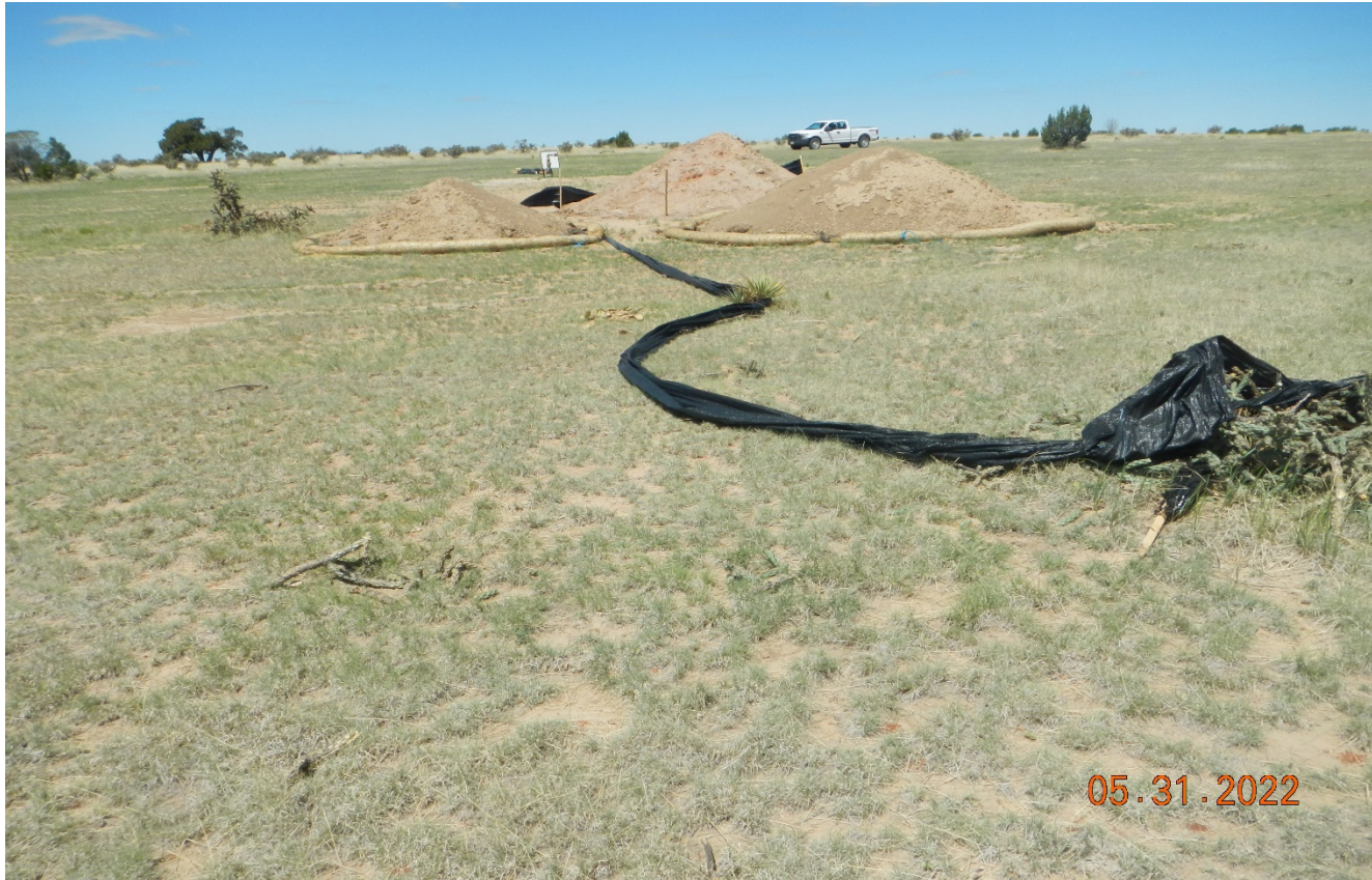
Photo 6. The silt fence is strung across the location.
