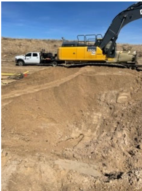
6 – 70 Ranch 32-27 – PWV excavation; looking east. Circular fiberglass vault removed prior to arrival
