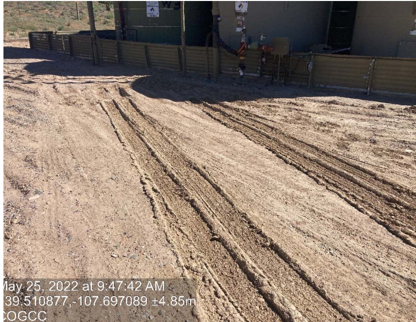
Lack of stabilization/ compaction/ degradation
