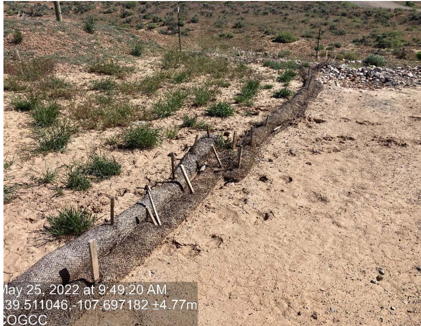
BMP's Failing and debris
