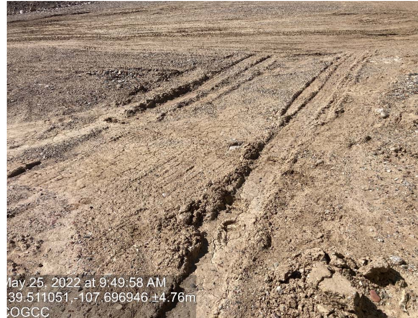
Lack of stabilization/ compaction/ degradation
