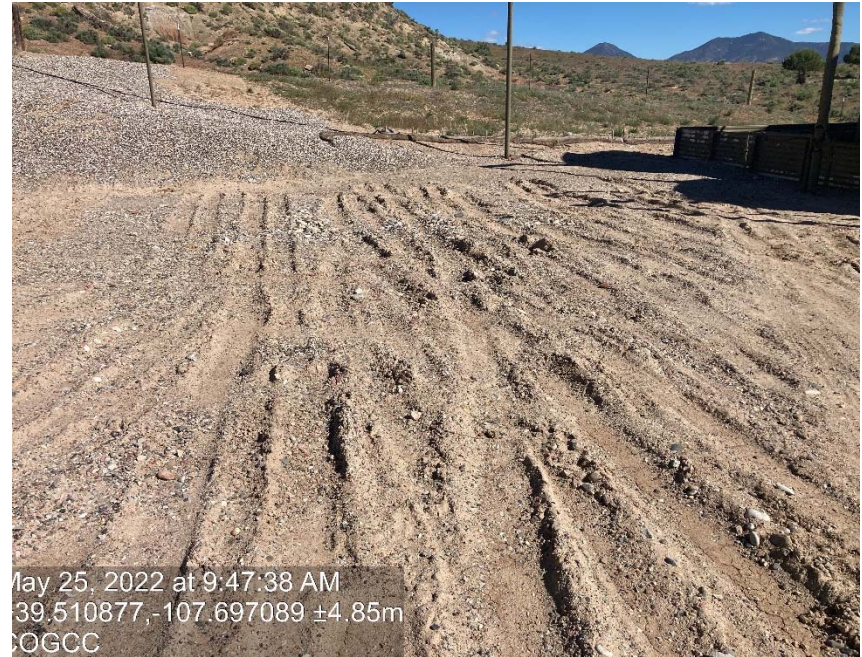
Recent photo of Lack of stabilization/ compaction/ degradation
