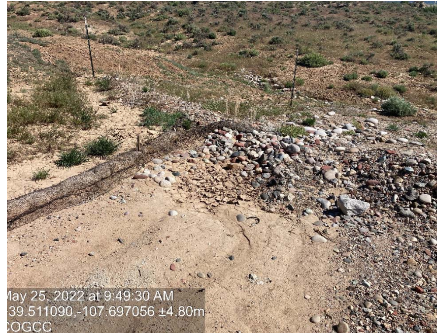
BMP's Failing and debris
