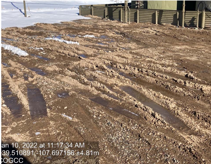
Previous inspection of Lack of stabilization/ compaction/ degradation
