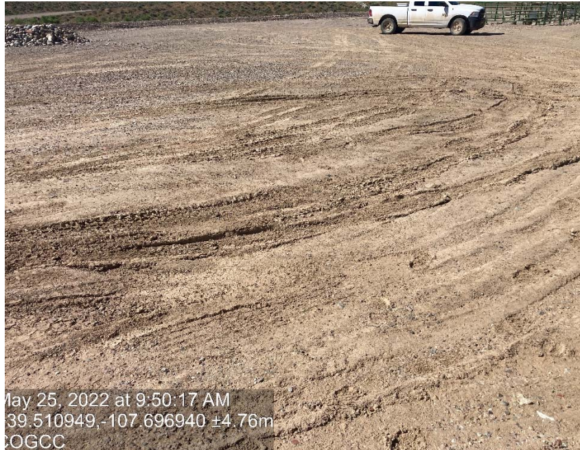
Lack of stabilization/ compaction/ degradation
