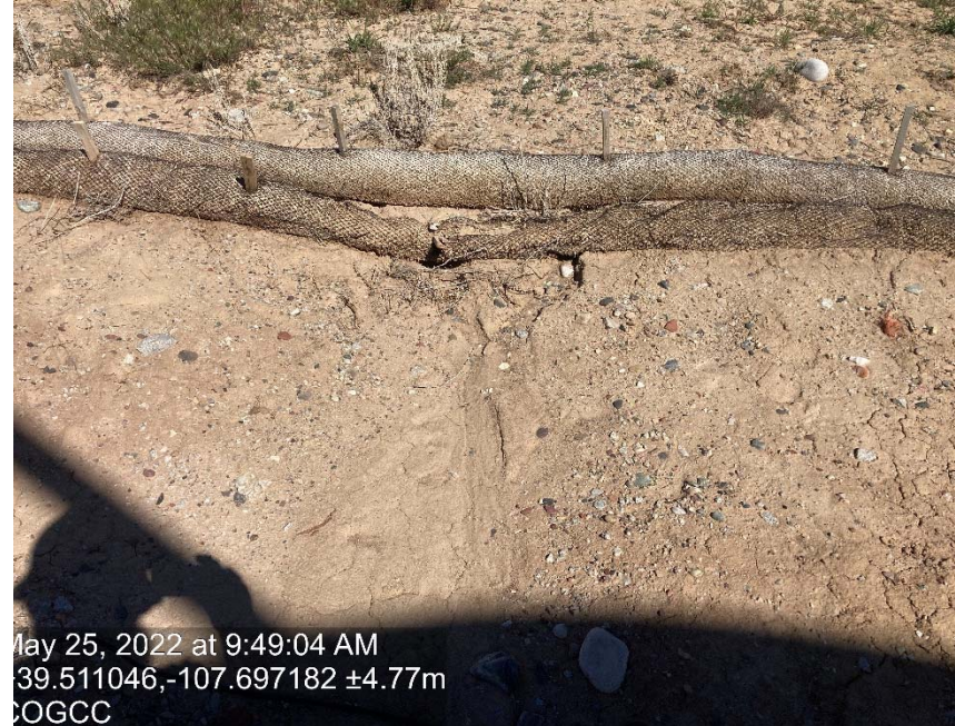
BMP's Failing and debris
