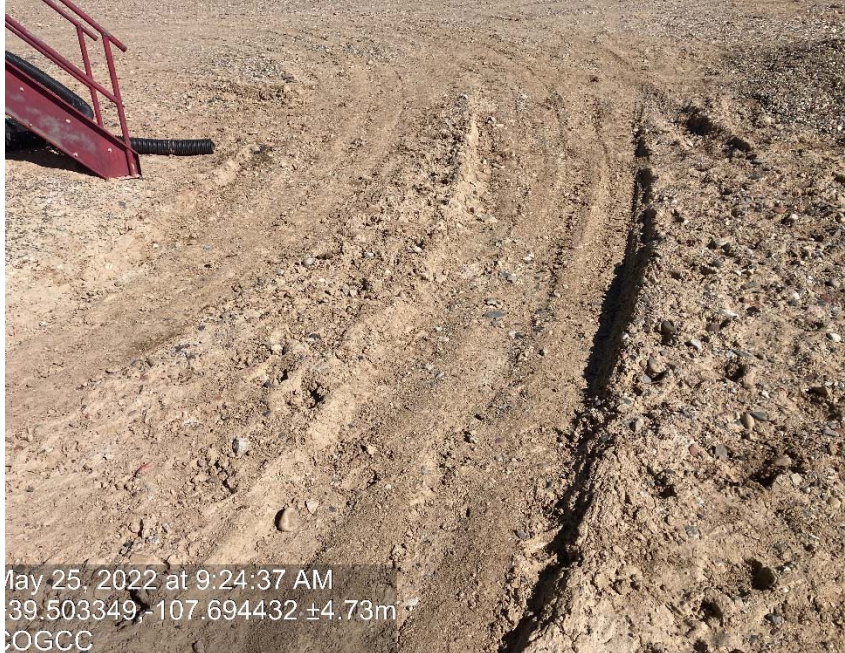
Lack of stabilization/ compaction/ degradation
