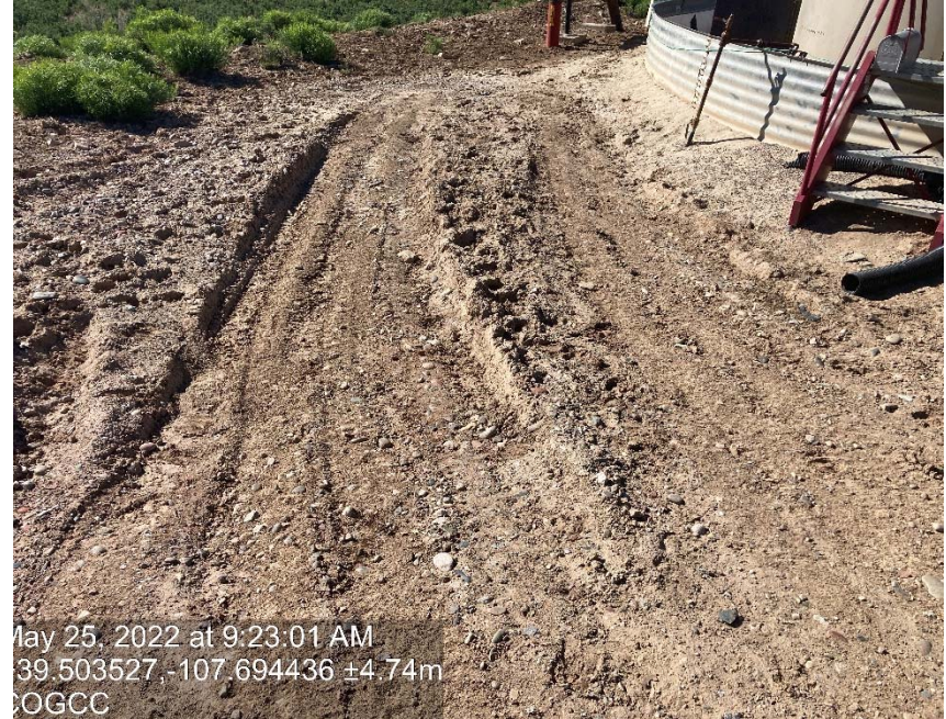
Lack of stabilization/ compaction/ degradation
