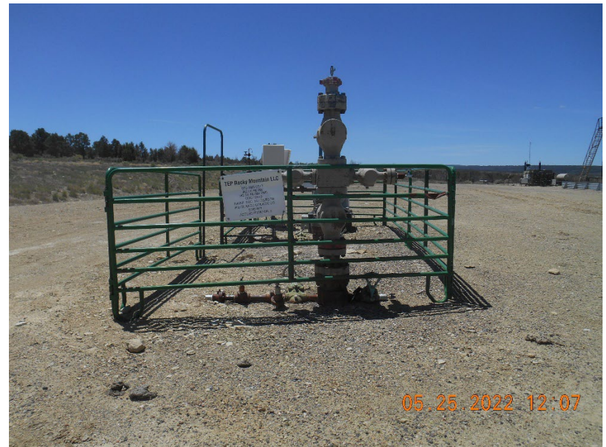
Temporarily abandoned Injection wellhead & Producing wellhead with chemical injection.
