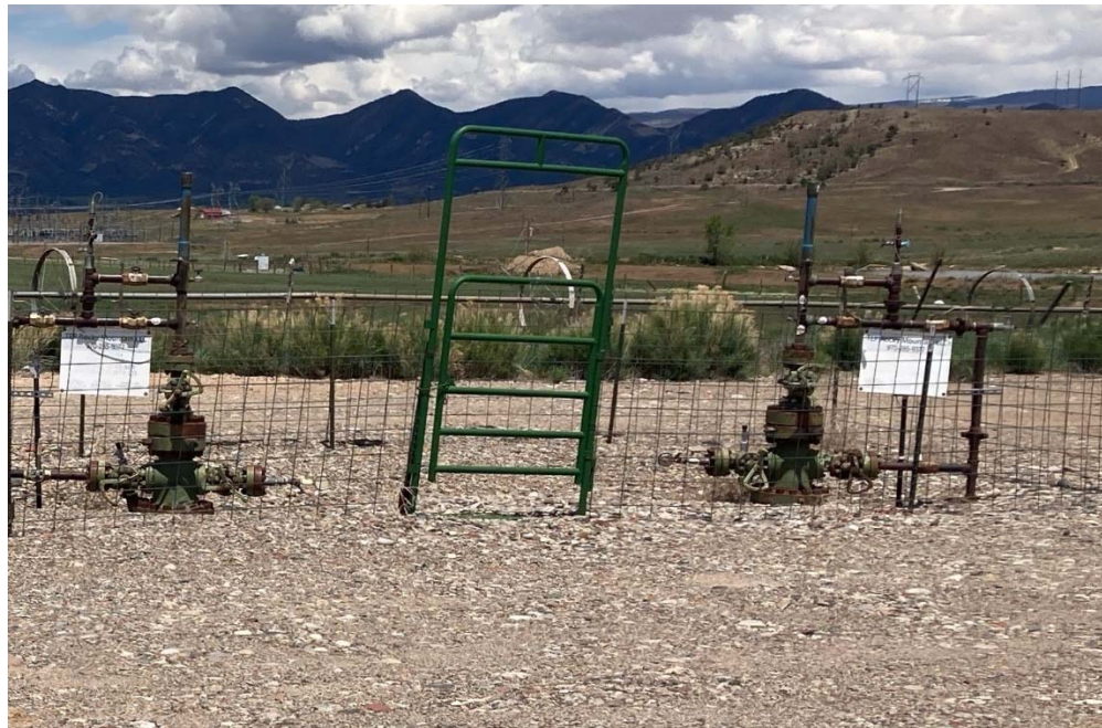
Well head signs are faded and illegible
