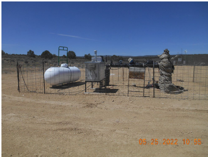
Injection wellhead & line heater
