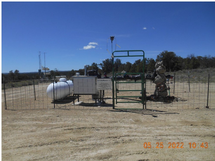
Injection wellhead & line heater
