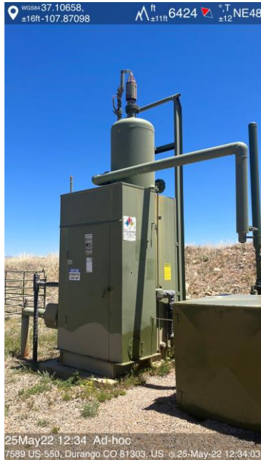
IMG 15 Separator with vent screen
