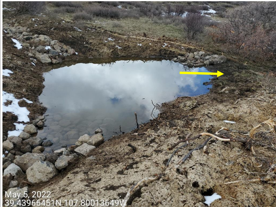
Photo 6: Photo taken from the sediment trap on the northwest end of the Location. Outlet inadequate in side; stormwater runoff discharging to areas around the trap's outlet.
