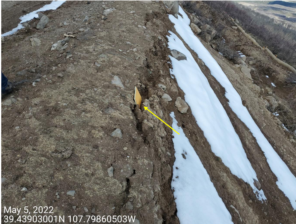
Photo 10: Photo taken from the fill slopes on the north end of the Location. Photo shows large crack forming on the slopes. Notebook for reference; slopes unstabilized and appear to be sloughing.
