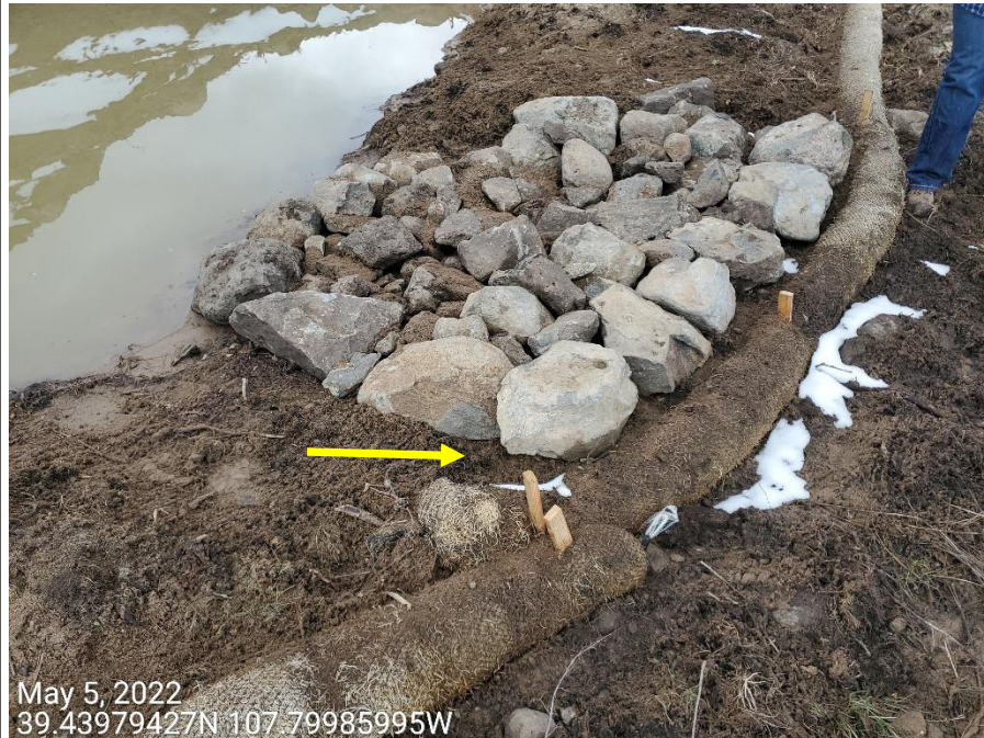
Photo 5: Photo taken from the sediment trap on the north end of the Location. Outlet inadequate; stormwater runoff discharging to areas around the trap's outlet, resulting in degradation to the control. Photo also shows sediment deposition on top of the straw wattle leading offsite.
