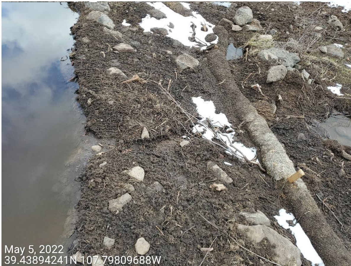
Photo 3: Continued from photo 1. Photo a second example of the sediment trap where an outlet has not been constructed, but where stormwater is discharging, resulting in erosion degradation and sediment transport. Photo left shows water has cut beneath the straw wattle.
