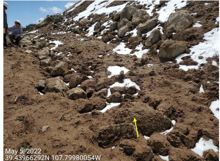
Photo 8: Continued from photo 7. Photos example shows sediment deposition as a result of the erosion degradation from the unstabilized fill slopes
