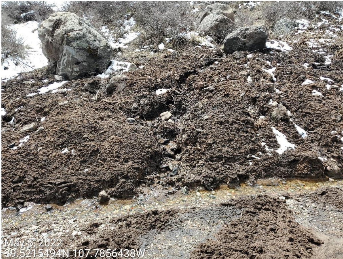
Photo 13: Photo example showing BMPs at the topsoil along the access road have not been maintained.
