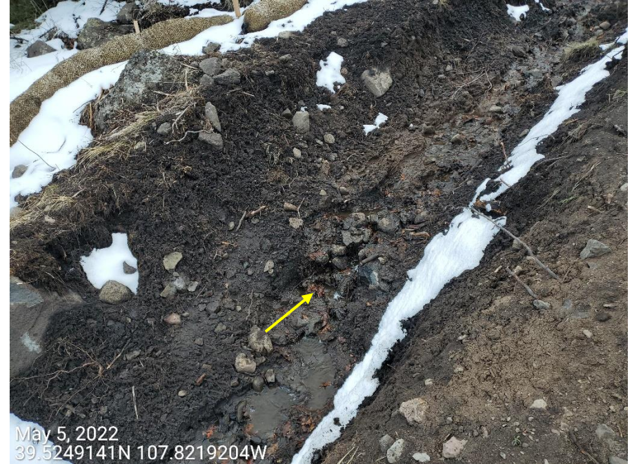
Photo 9: Photos example showing the perimeter stormwater diversion ditch of the Location; majority of the ditch has been constructed with vertical slopes and unconsolidated soils; this is not per good engineering practices. Photo right shows stormwater degradation within the control, and unsoncolidated “fine soils” have eroded away.
