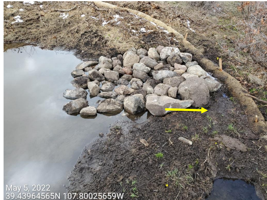
Photo 6: Photo taken from the sediment trap on the northwest end of the Location. Outlet inadequate in side; stormwater runoff discharging to areas around the trap's outlet.
