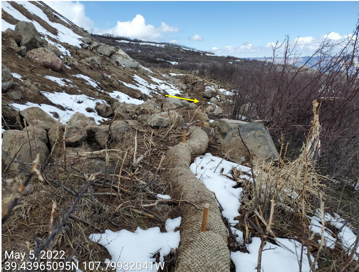
Photo 11: Photo example showing low points within the ditch along the north end of the Location, where stormwater is discharging from, rather than flowing into the northwestern sediment traps.
