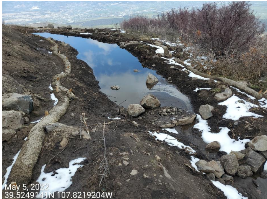
Photo 1: Photos taken from the sediment trap on the northeast end of the Location. Photo right shows sediment deposition due to unstabilize soils within the stormwater ditch.
