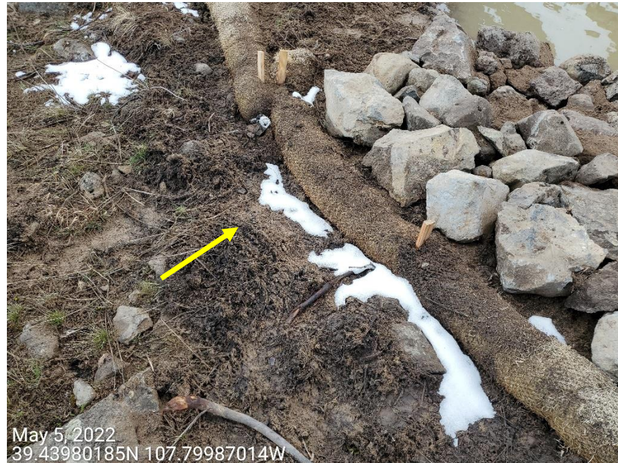
Photo 5: Photo taken from the sediment trap on the north end of the Location. Outlet inadequate; stormwater runoff discharging to areas around the trap's outlet, resulting in degradation to the control. Photo also shows sediment deposition on top of the straw wattle leading offsite.
