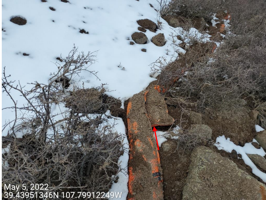
Photo 9: Photos example shows sediment deposition as a result of the erosion degradation from the unstabilized fill slopes. Photo right also shows remnants of the hydromulch that was previously applied, and is now covered with sediment from the fill slopes.
