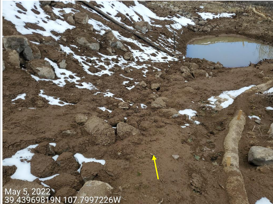
Photo 8: Continued from photo 7. Photos example shows sediment deposition as a result of the erosion degradation from the unstabilized fill slopes
