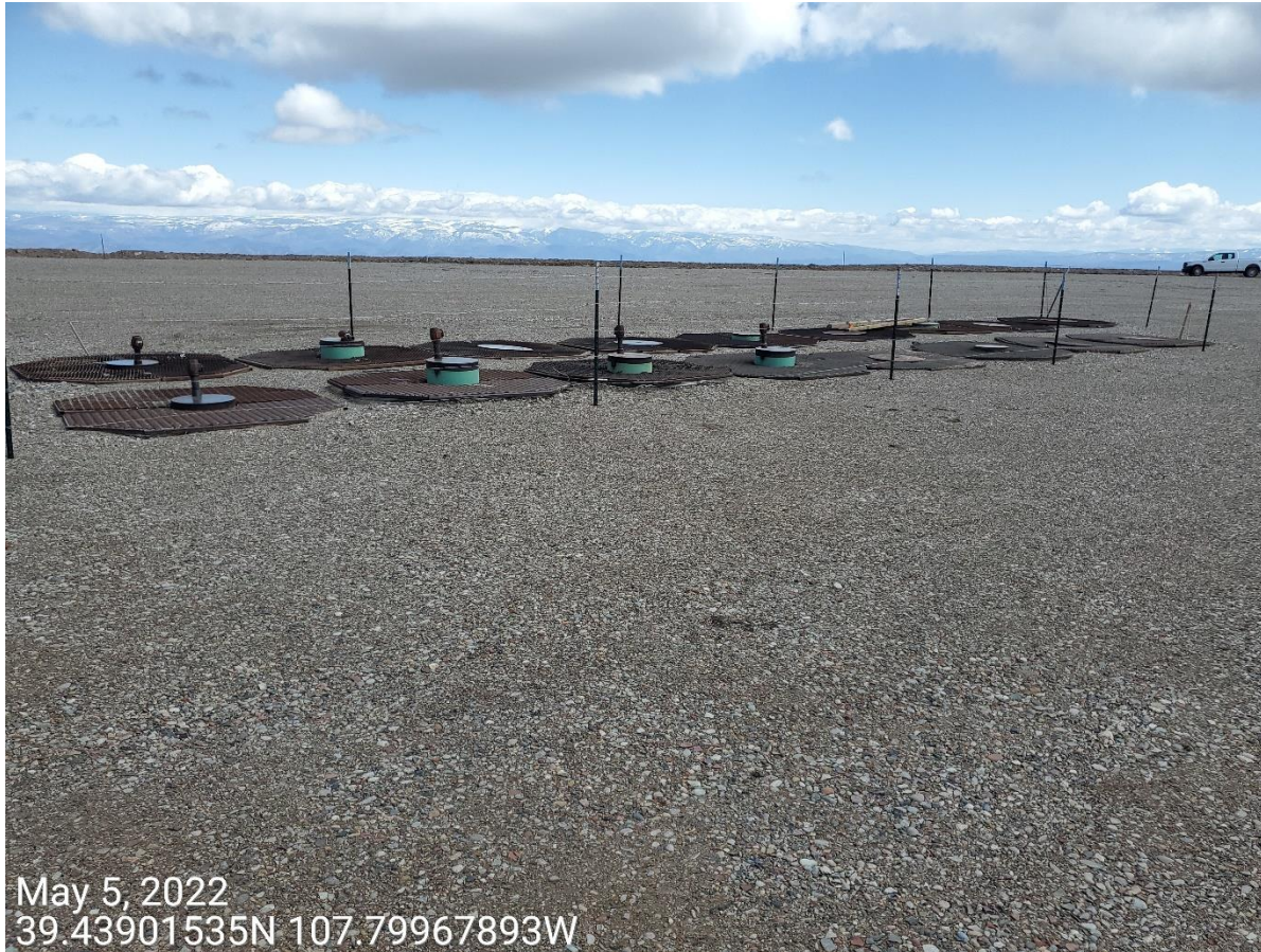
Photo 16: Photo shows conductor settings on Location; wells have not been drilled.
