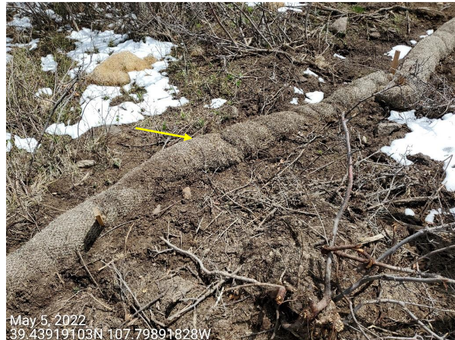
Photo 12: Continued from photo 11. Photo example showing low points within the ditch along the north end of the Location, where stormwater is discharging from, rather than flowing into the northwestern sediment traps.
