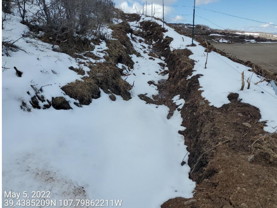
Photo 9: Photos example showing the perimeter stormwater diversion ditch of the Location; majority of the ditch has been constructed with vertical slopes and unconsolidated soils; this is not per good engineering practices. Photo right shows stormwater degradation within the control, and unsoncolidated “fine soils” have eroded away.
