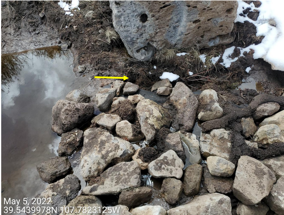
Photo 4: Photo taken from the sediment trap on the southwest end of the Location. Outlet inadequate; stormwater runoff discharging to areas around the trap's outlet, resulting in degradation to the control.
