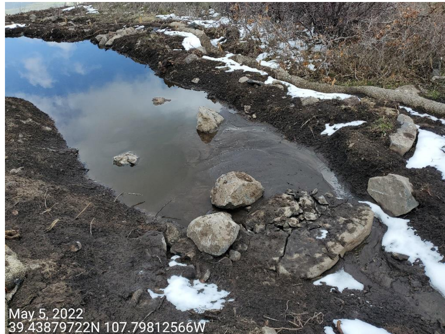
Photo 1: Photos taken from the sediment trap on the northeast end of the Location. Photo right shows sediment deposition due to unstabilize soils within the stormwater ditch.
