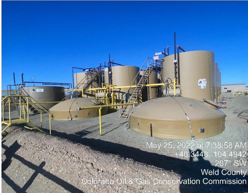
Photo #9 Missing Pit Capacity/ Placard Labels
