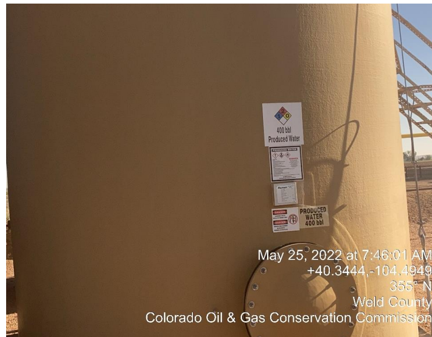
Photo #16 Inaccurate capacity label
