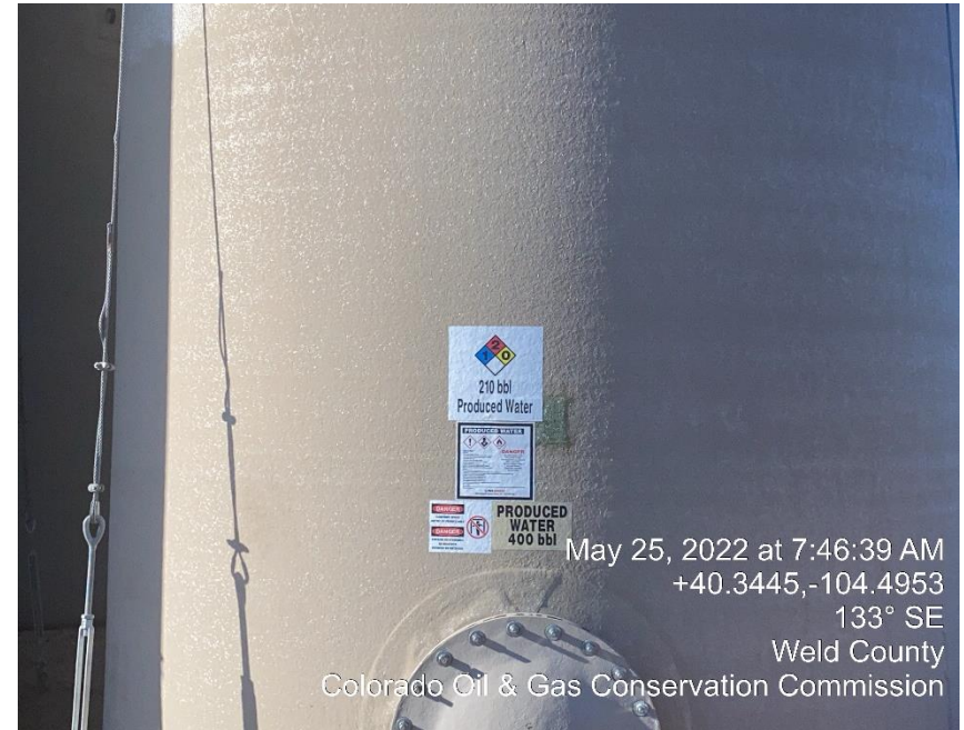
Photo #18 Inaccurate capacity label
