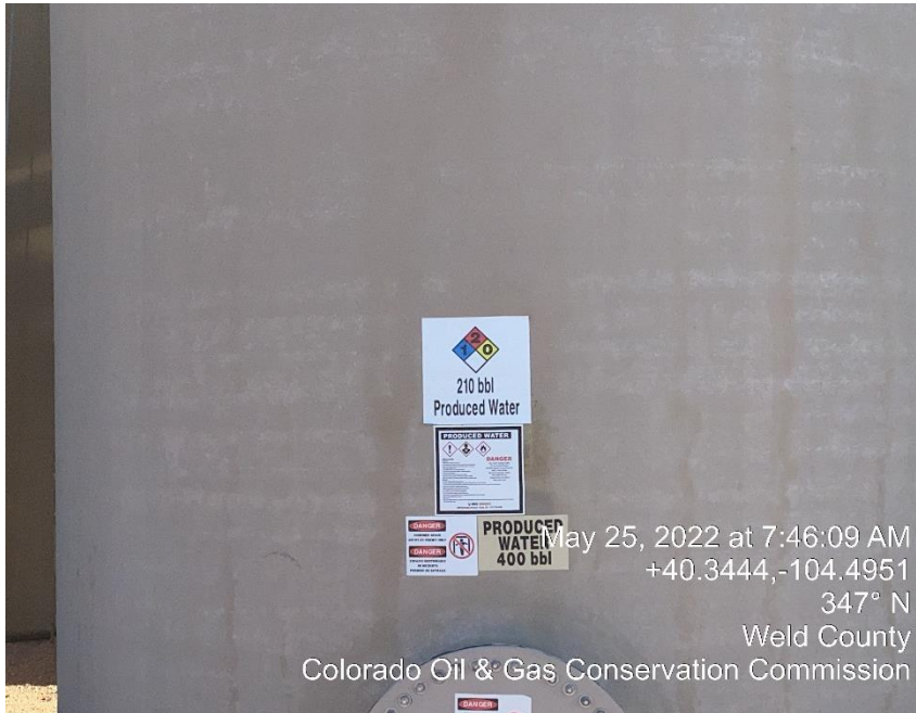
Photo #17 Inaccurate capacity label
