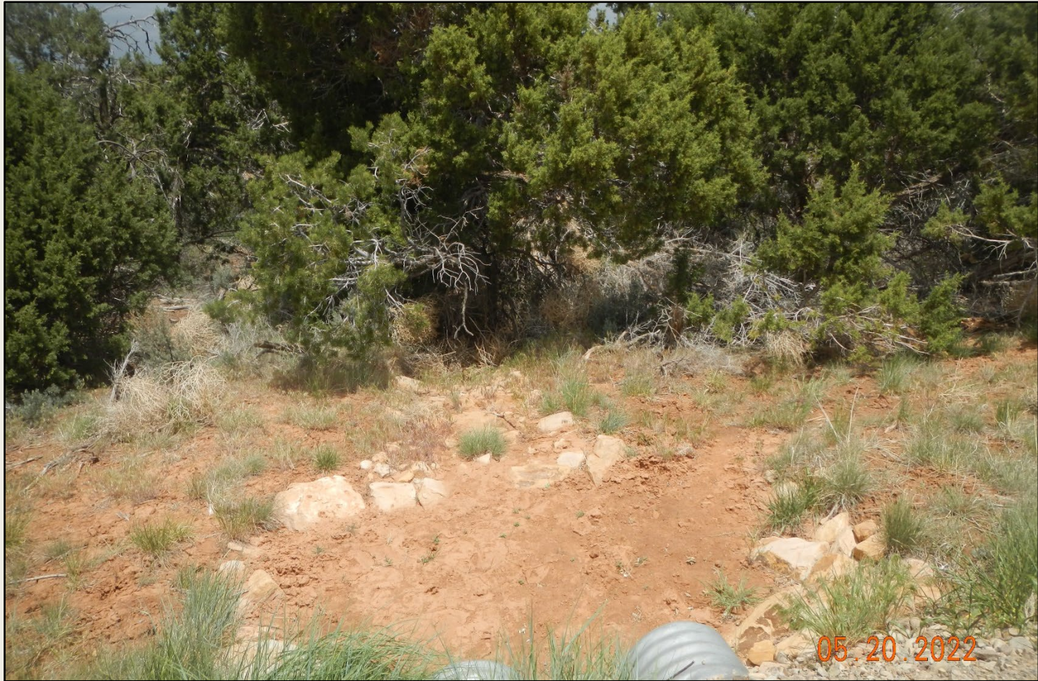
Photo 5. View of another culvert outlet along the access road that is full of sediment and is not an adequate long-term stabilization measure.
