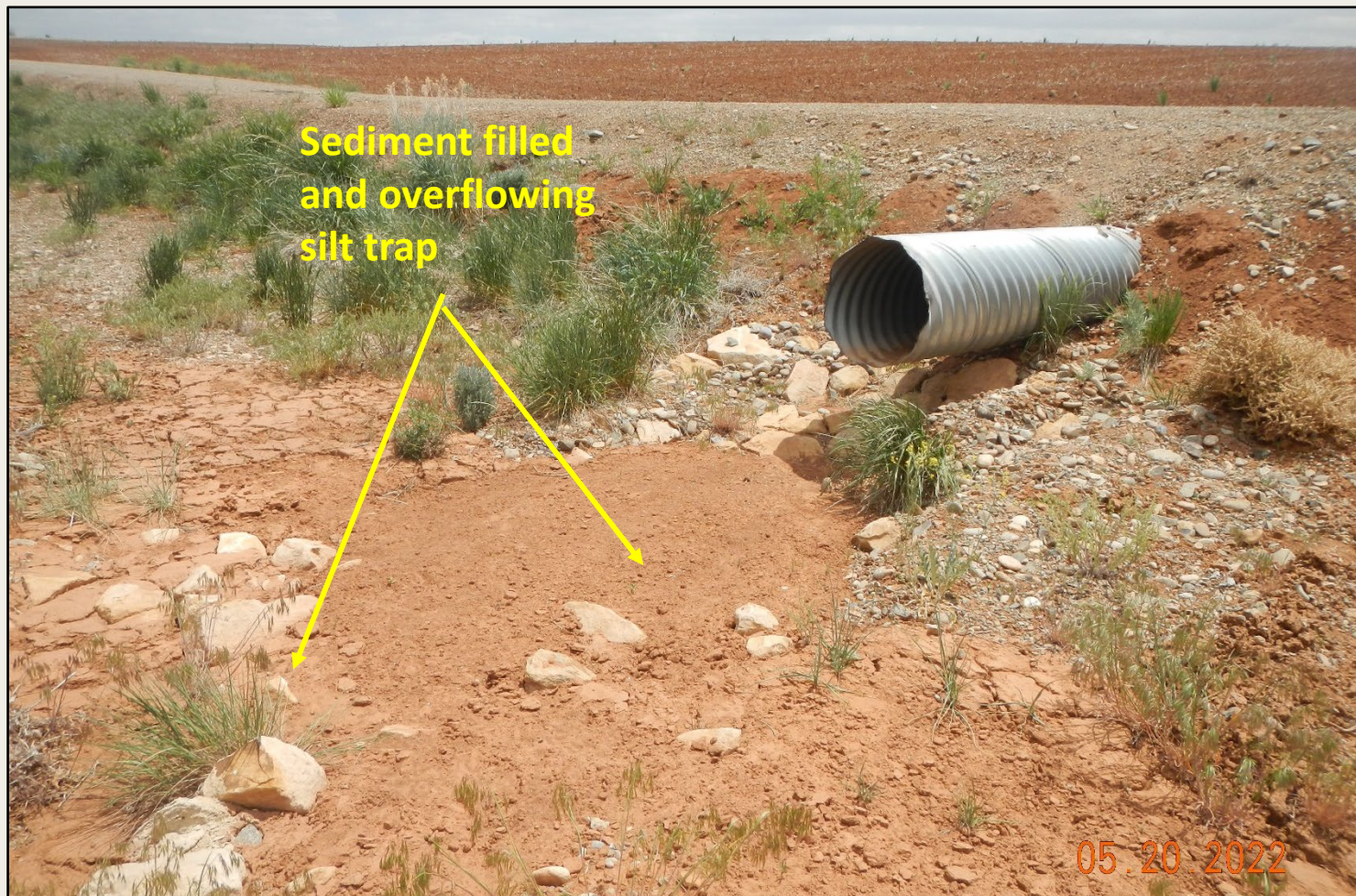
Photo 3. View of culvert outlet along the access road where sediment is accumulated and is overflowing silt trap off and flowing offsite.
