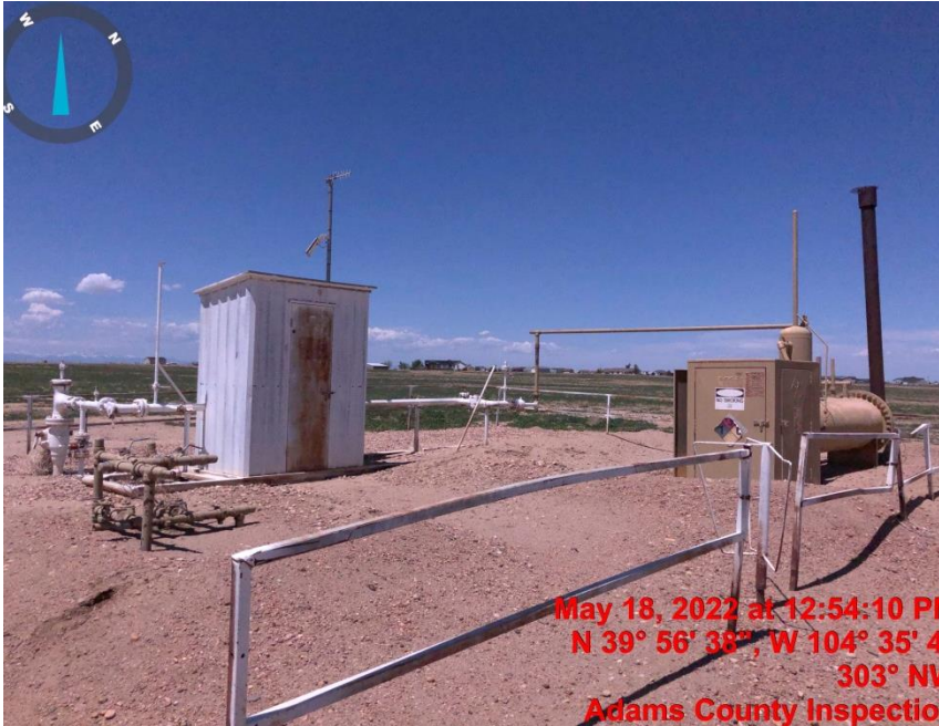
Photo#5 Separator and Gas Meter
