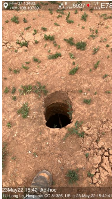
IMG 05 Unfilled Mousehole
