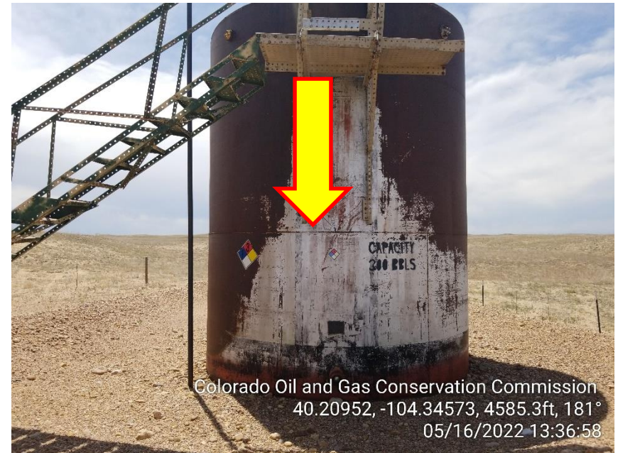
Photo 16 – Content Label Missing
