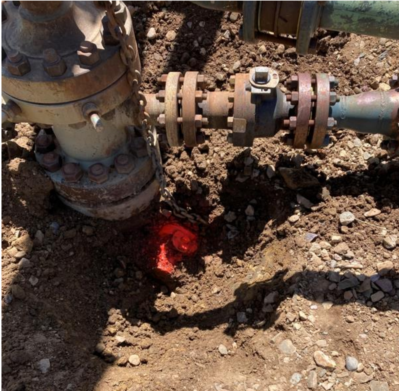
PHOTO 1: THE BRADENHEAD HAS BEEN MADE ACCESSABLE AND VISIBLE TO ALLOW FOR INSPECTION
