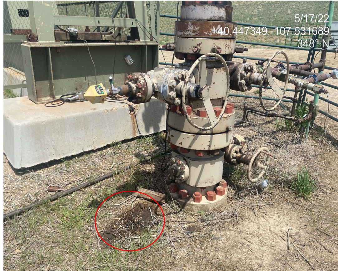
Photo 4. Photo taken from the wellhead shows stained soils.
