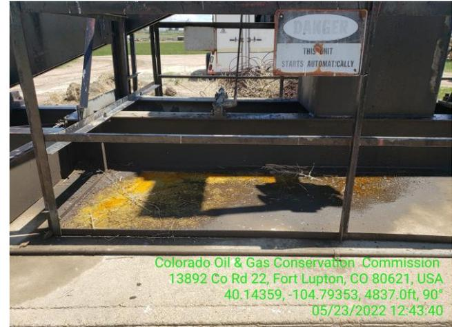
Photo 9 Stained concrete due to leaking seal.
