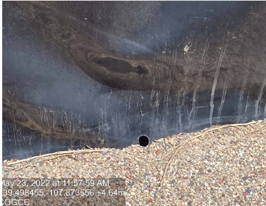
Hole in containment
