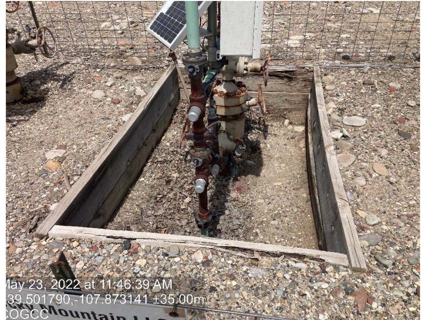
Well head cellar missing wildlife egress
