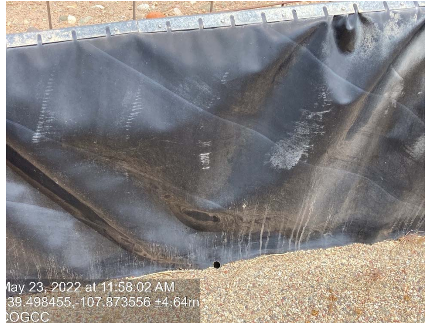
Hole in containment
