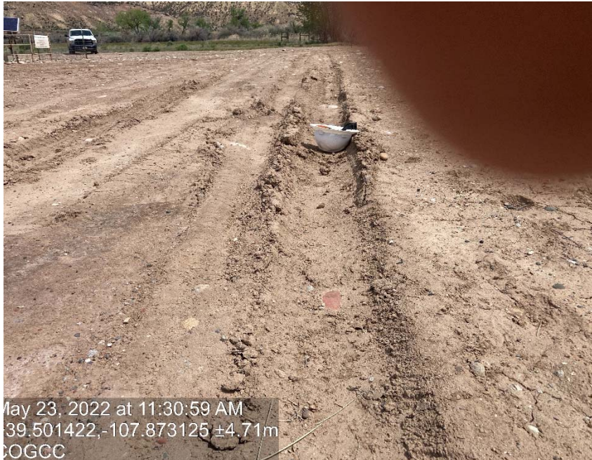
Lack of stabilization/compaction
