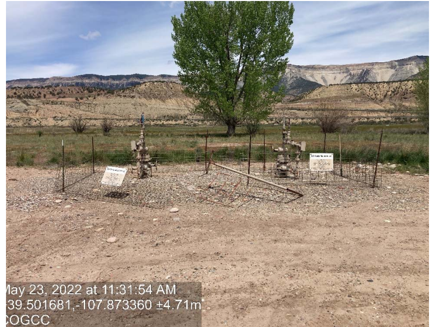
Well heads gate and fence falling down
