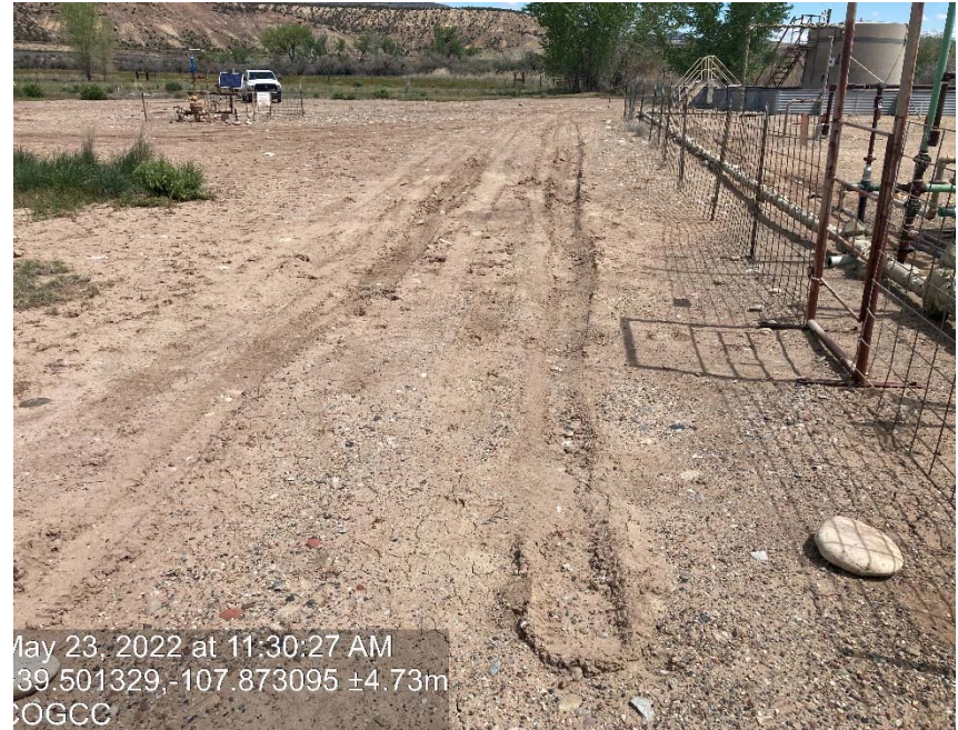
Lack of stabilization/compaction
