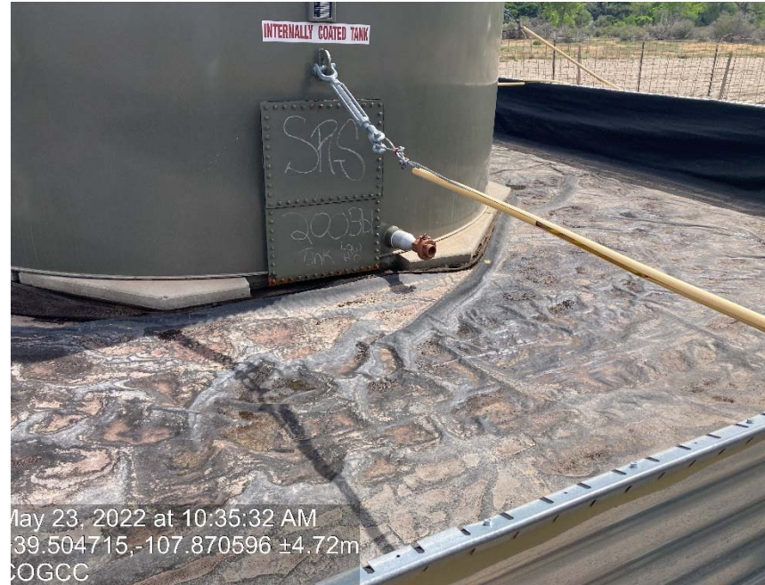
Valve missing cap/plug
