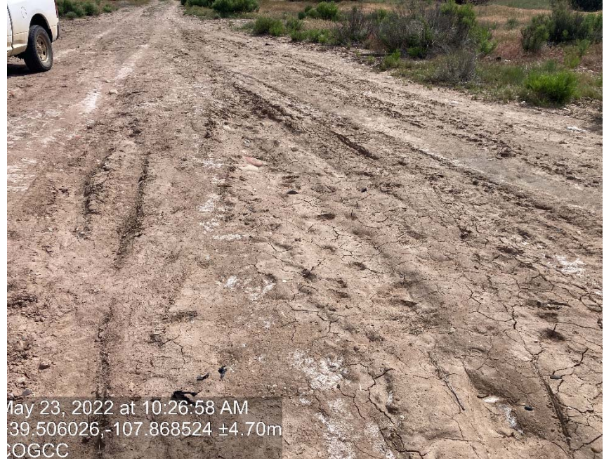
Lack of stabilization/compaction
