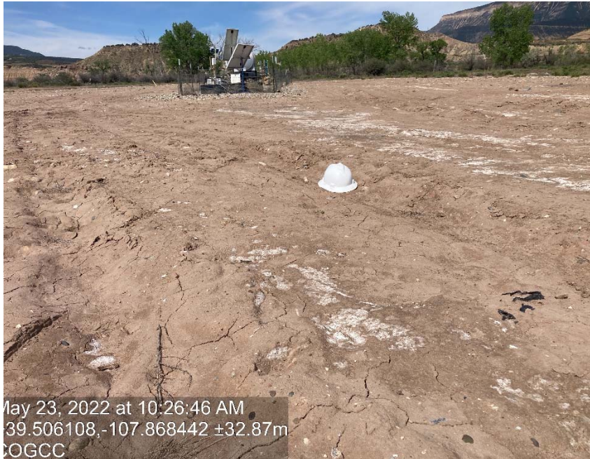
Lack of stabilization/compaction
