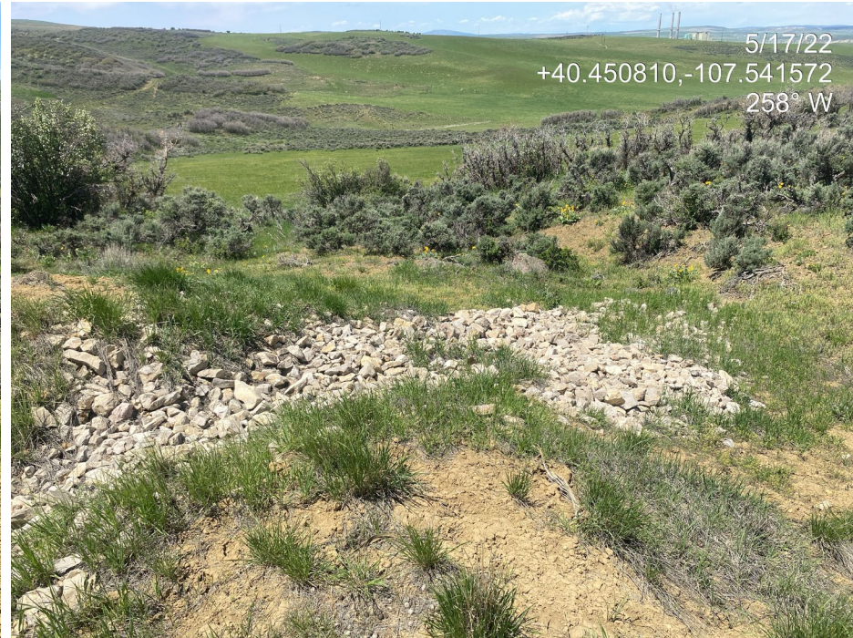
Photo 9. Photo taken from the southwest of the Location shows a rip-rap lined stormwater outlet. The BMP appears to be functioning to manage stormwater on the Location in conjunction with perennial plant establishment.
