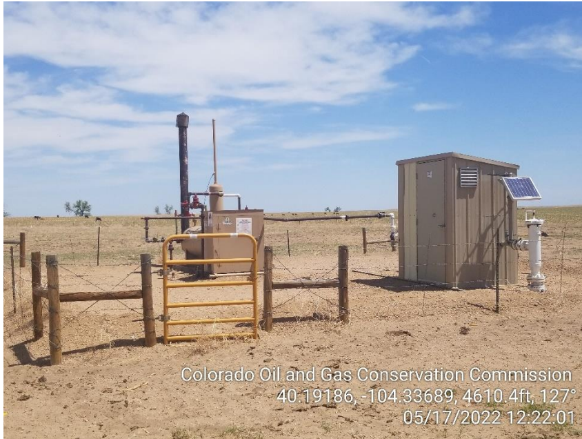
Photo 5 – Separator and Gas Meter
