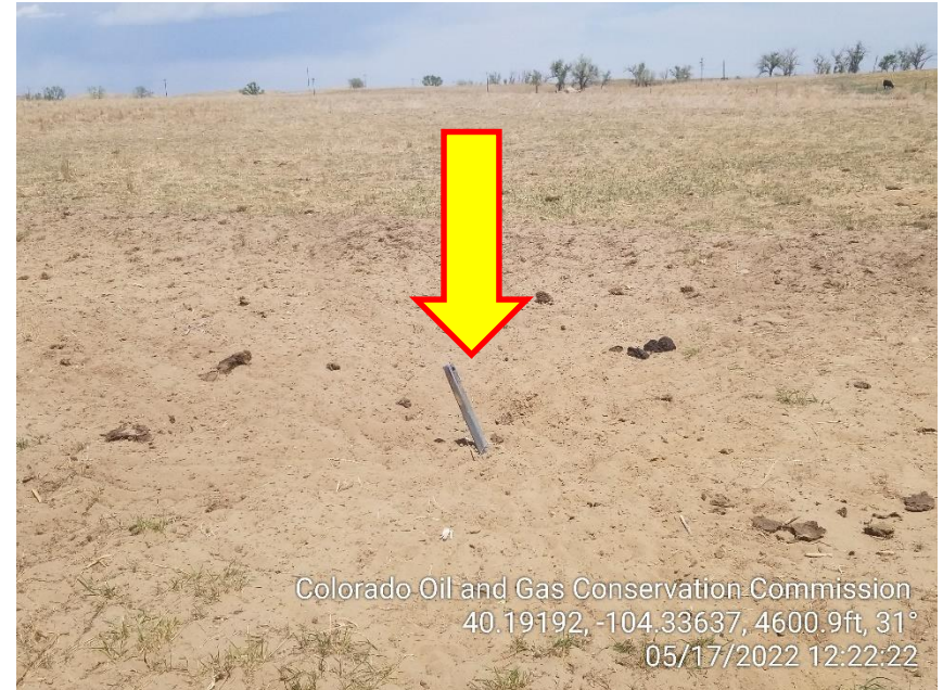
Photo 6 – NE Deadman Anchor – Not Marked
