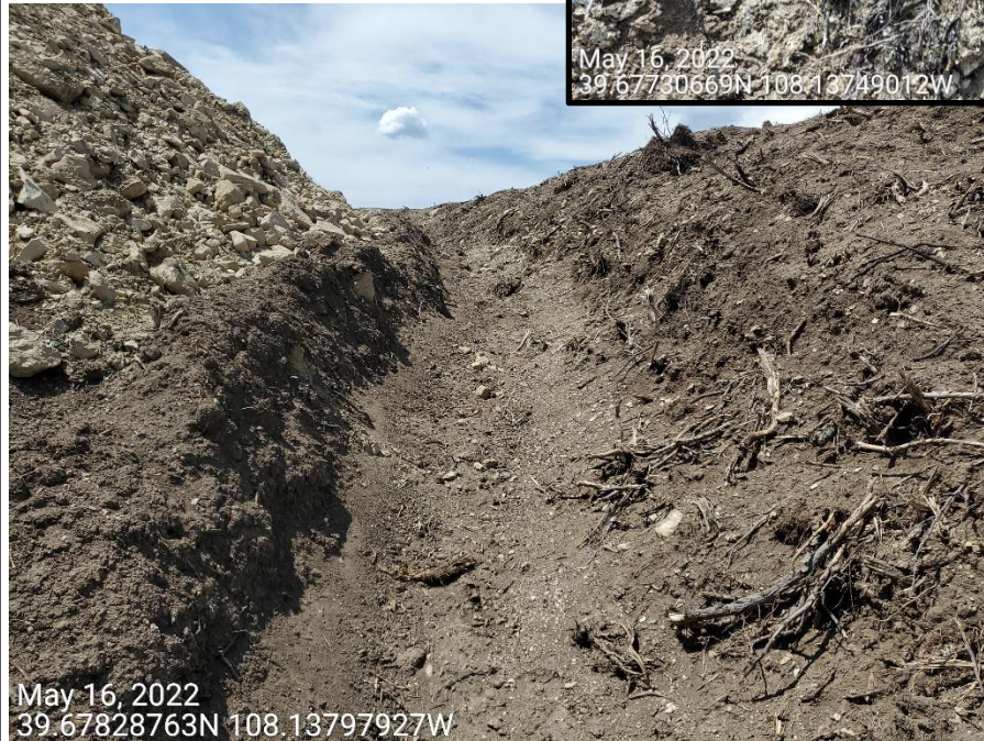
Photo 3: See comments under photo 2. Photo also shows loose soils within the ditch, unstabilized slopes within the ditch BMP and along the topsoil stockpile, and that topsoil is evident within slopes of the ditch. BMPs to protect the soil stockpile remains inadequate.
