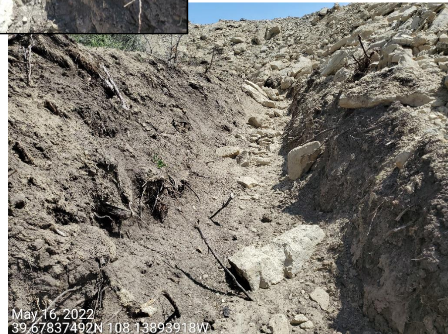
Photo 4: See comments under photo 2. Photo also shows loose soils within the ditch, unstabilized slopes within the ditch BMP and along the topsoil stockpile, and that topsoil is evident within slopes of the ditch. BMPs to protect the soil stockpile remains inadequate.
