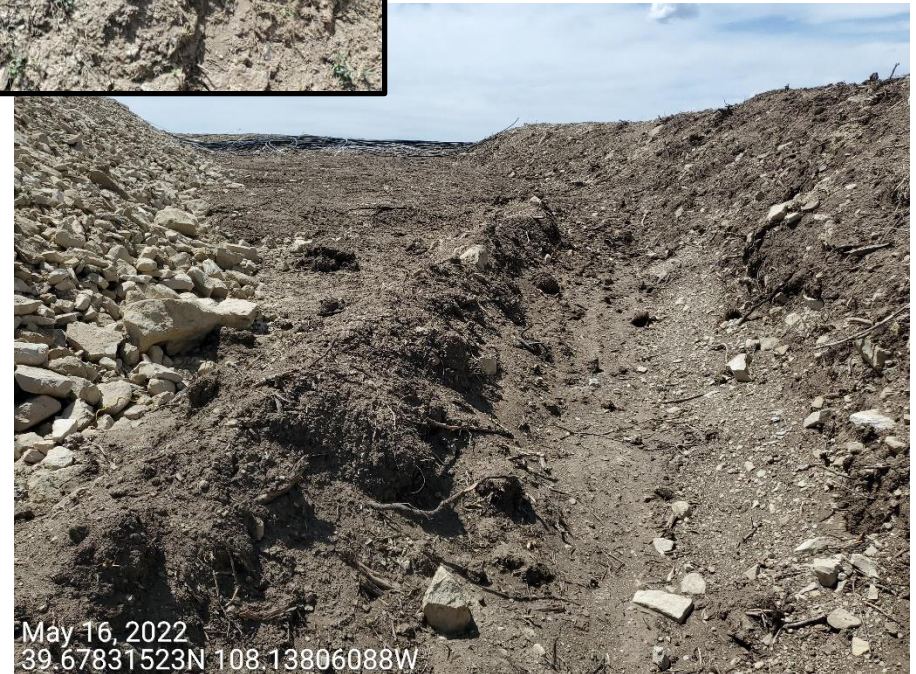
Photo 3: See comments under photo 2. Photo also shows loose soils within the ditch, unstabilized slopes within the ditch BMP and along the topsoil stockpile, and that topsoil is evident within slopes of the ditch. BMPs to protect the soil stockpile remains inadequate.
