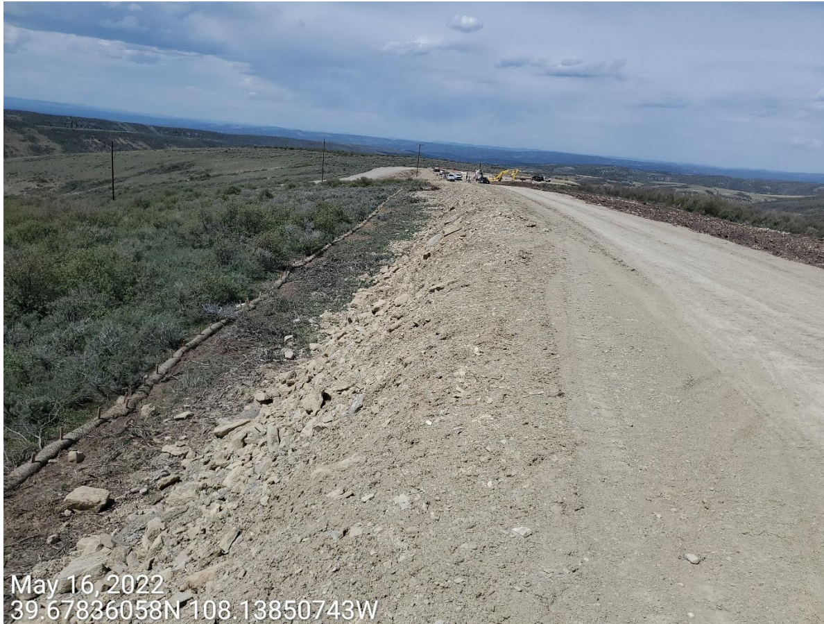
Photo 7: Photo taken from the north end of the Location, facing north. Photo shows access road that travels north to the BJU N26-496 Location. Inspection No. 696203136 documented that Operator failed to properly salvage/segregate and protect topsoil from areas beneath the access road disturbance.
