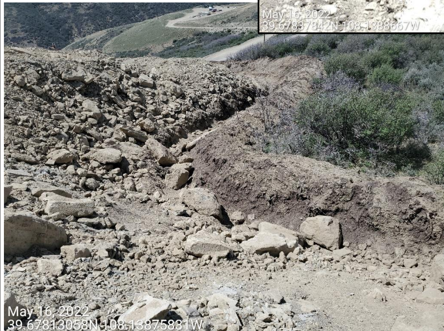
Photo 4: See comments under photo 2. Photo also shows loose soils within the ditch, unstabilized slopes within the ditch BMP and along the topsoil stockpile, and that topsoil is evident within slopes of the ditch. BMPs to protect the soil stockpile remains inadequate.
