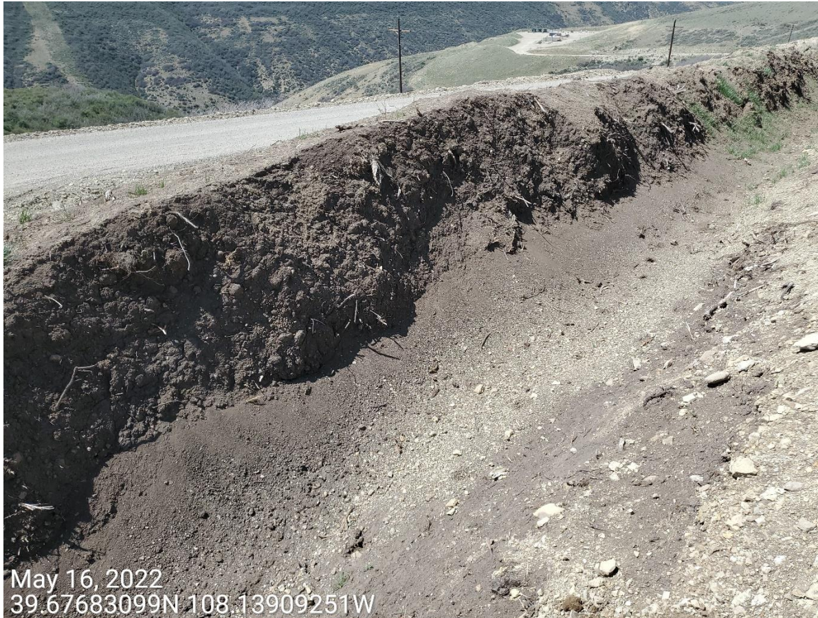
Photo 5: Photo example showing erosion occurring at the topsoil stockpile, and topsoil is being utilized as a stormwater control BMP.
