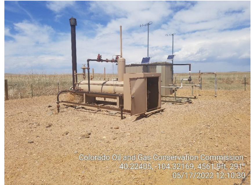
Photo 8 – Separator and Gas Meter
