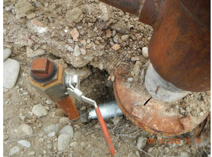
**Braden access installed. Gap in flange may not provide isolation.**
