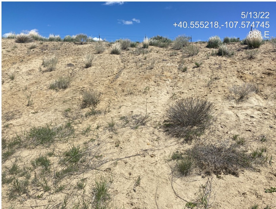
Photo 9. Photo taken from the north of the Location shows rill erosion occurring on the cut slope.
