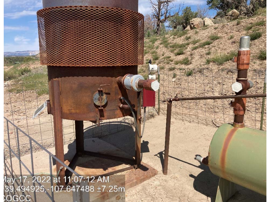
Stored equipment (ECD is disconnected from tanks and gas)
