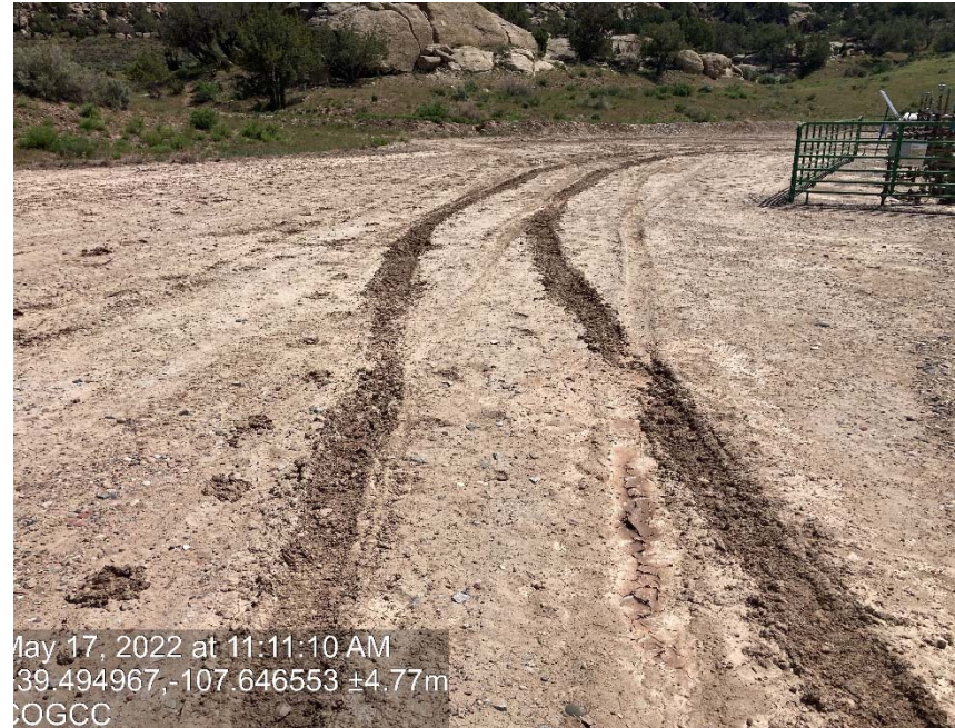
Lack of stabilization/compaction
