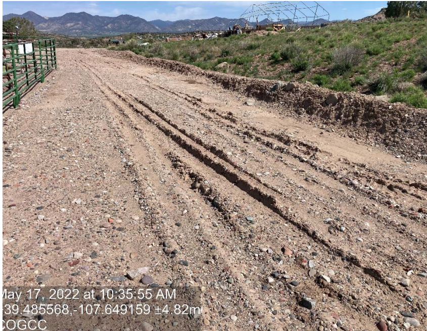
Lack of stabilization/compaction
