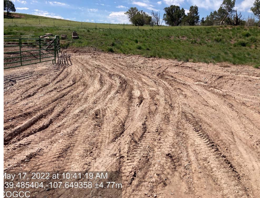
Lack of stabilization/compaction
