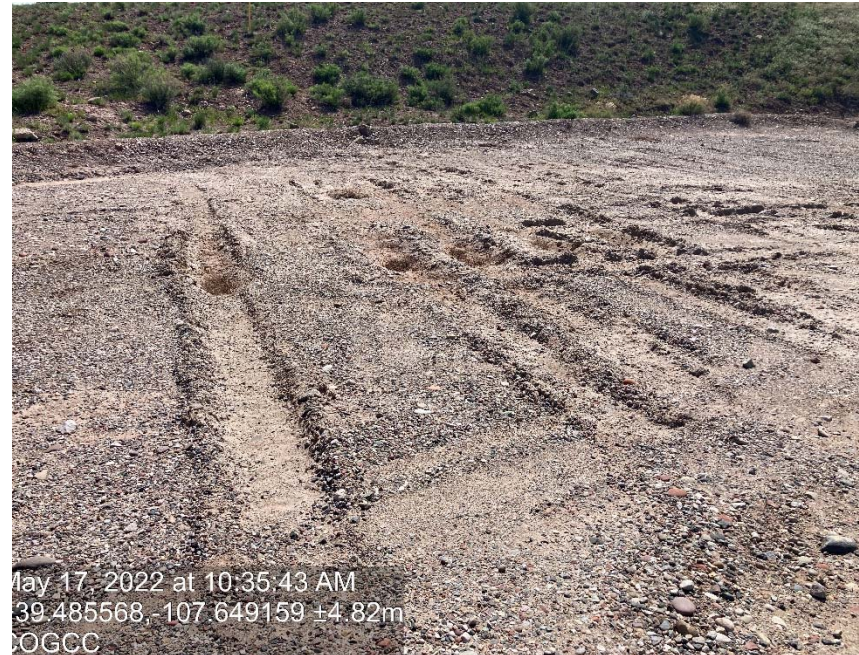
Lack of stabilization/compaction
