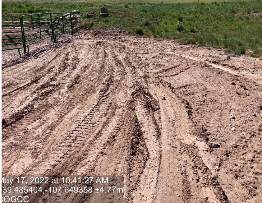
Lack of stabilization/compaction
