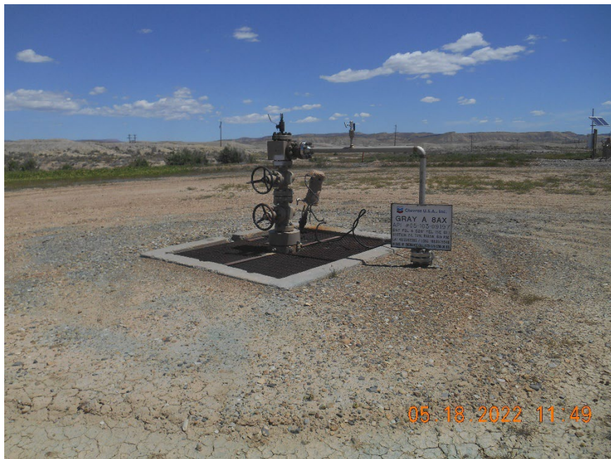
Injection wellhead.
