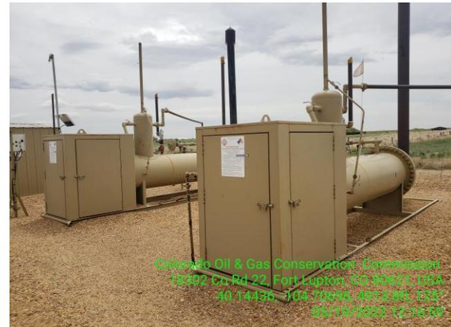
Photo 7 Gas Meter Run, Card indicates current calibration.
