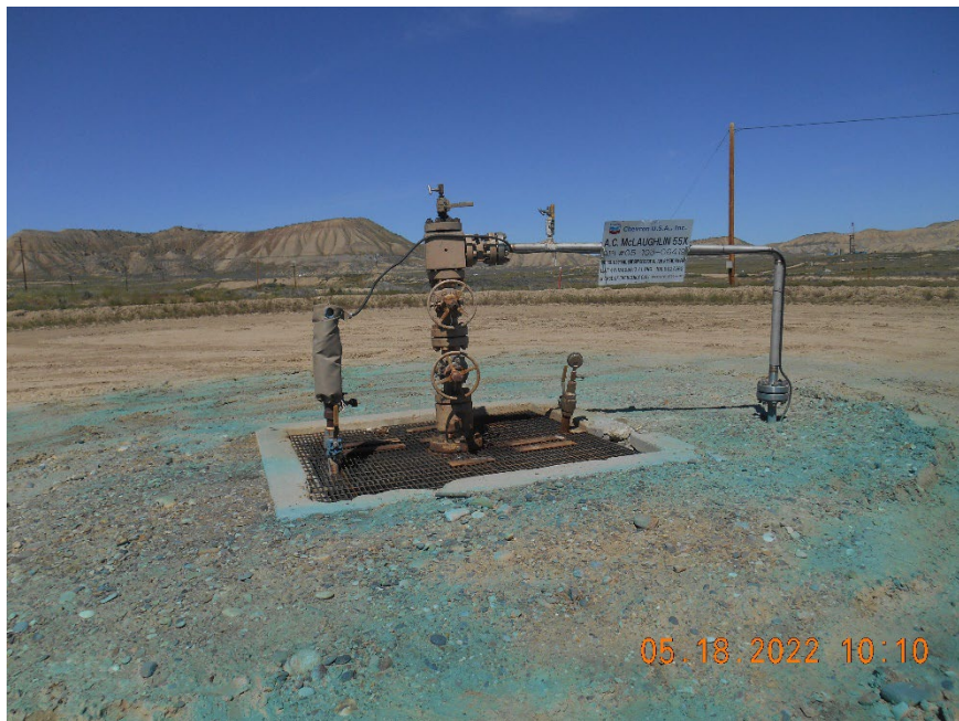
Injection wellhead
